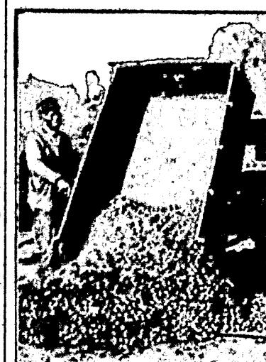
Truck Lead of Hot Bituminous Concrete Being Dumped Ready to Be Placed on Surface.
