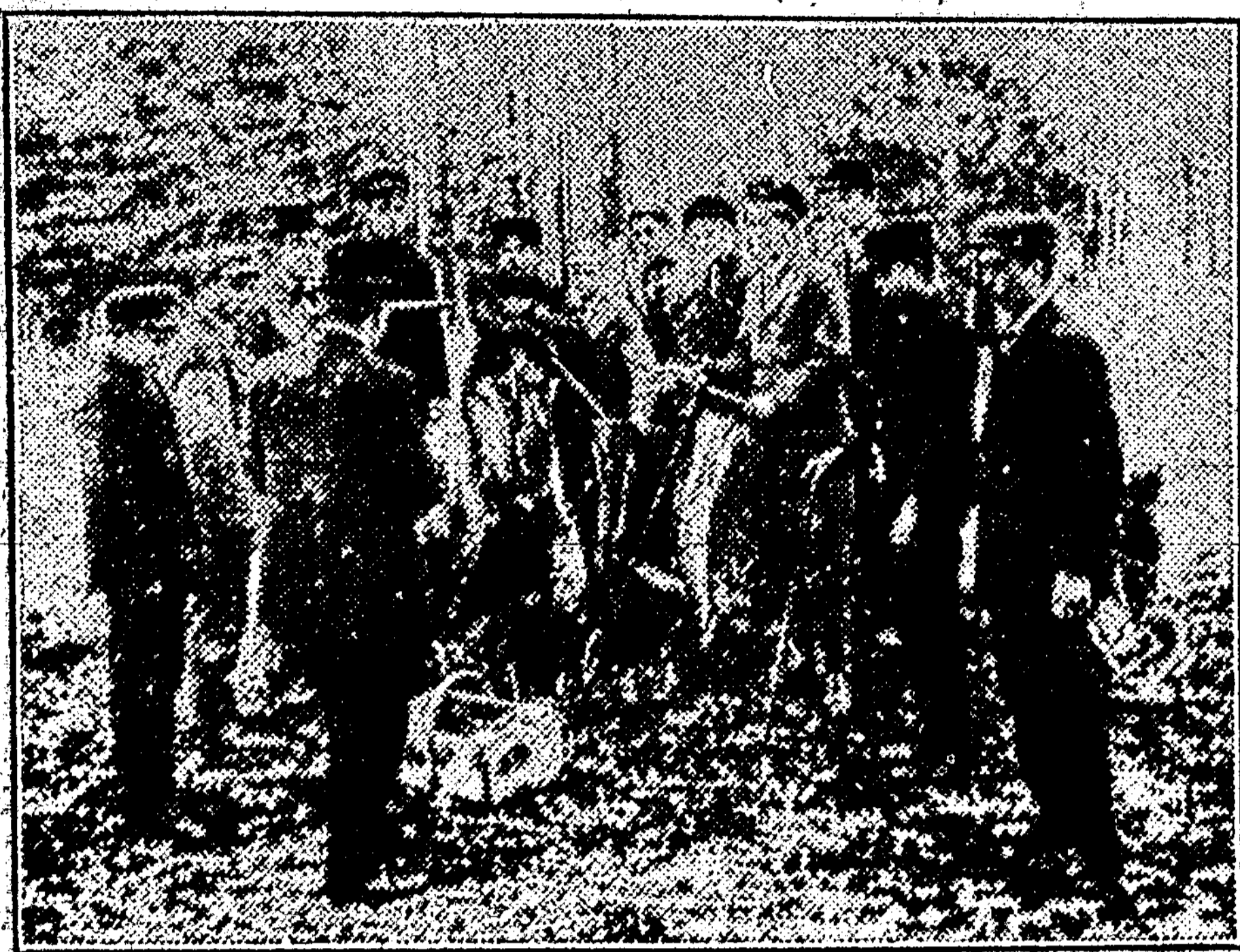
Students Removing Stumps With Dynamite.
