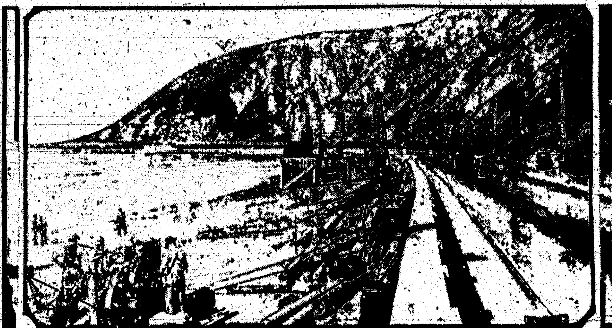
This view of the tidelands adjacent to the Coast highway near Santa Barbara, Calif., shows oil well drilling crews preparing to convert California's beautiful shoreline into a morass of derricks, kump holes and refuse dumps. This action on the part of oil prospectors has aroused the entire state to the need of preserving the beaches in their pristine beauty.
