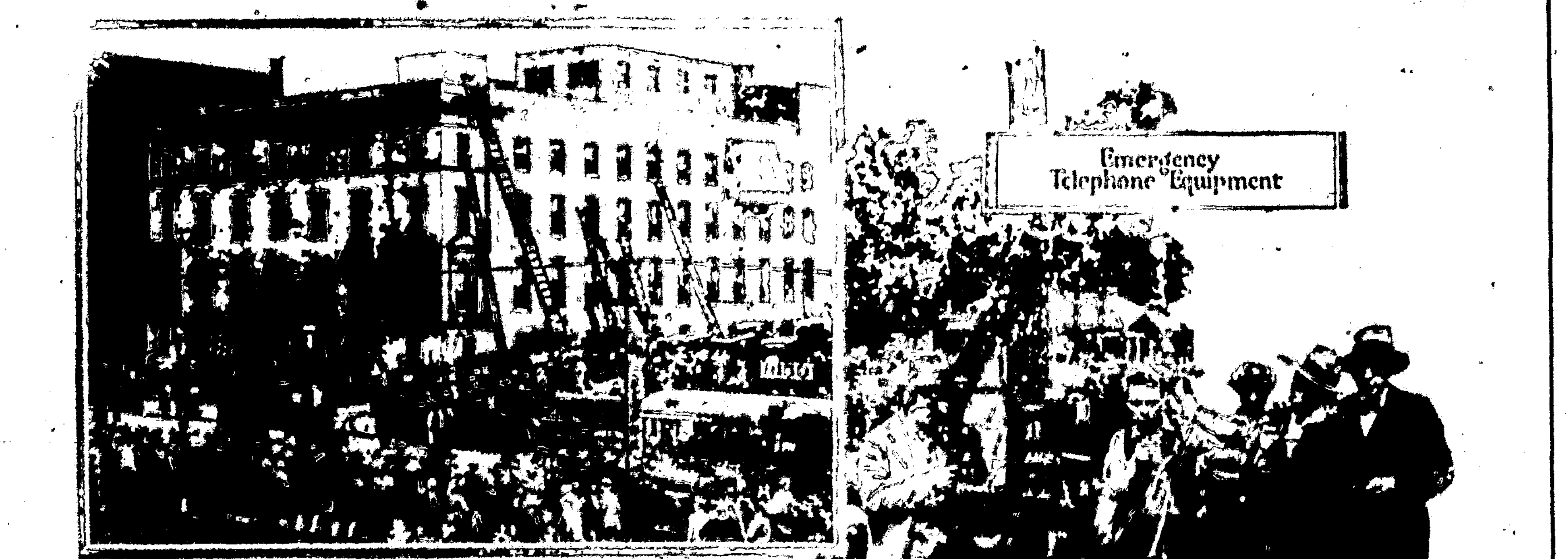
Cleveland Clinic Building During Rescue Work
