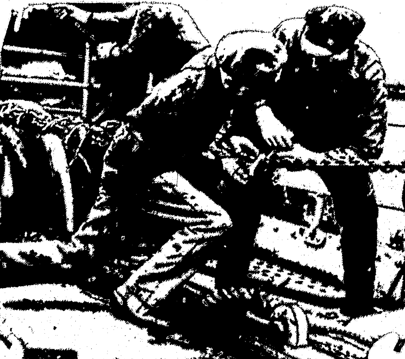
Several Atlantic cables were broken by the recent earthquake off the New England and Newfoundland coast. These men aboard the cable ship Cyrus Field are engaged in the difficult task of bringing up the broken ends and splicing them.
