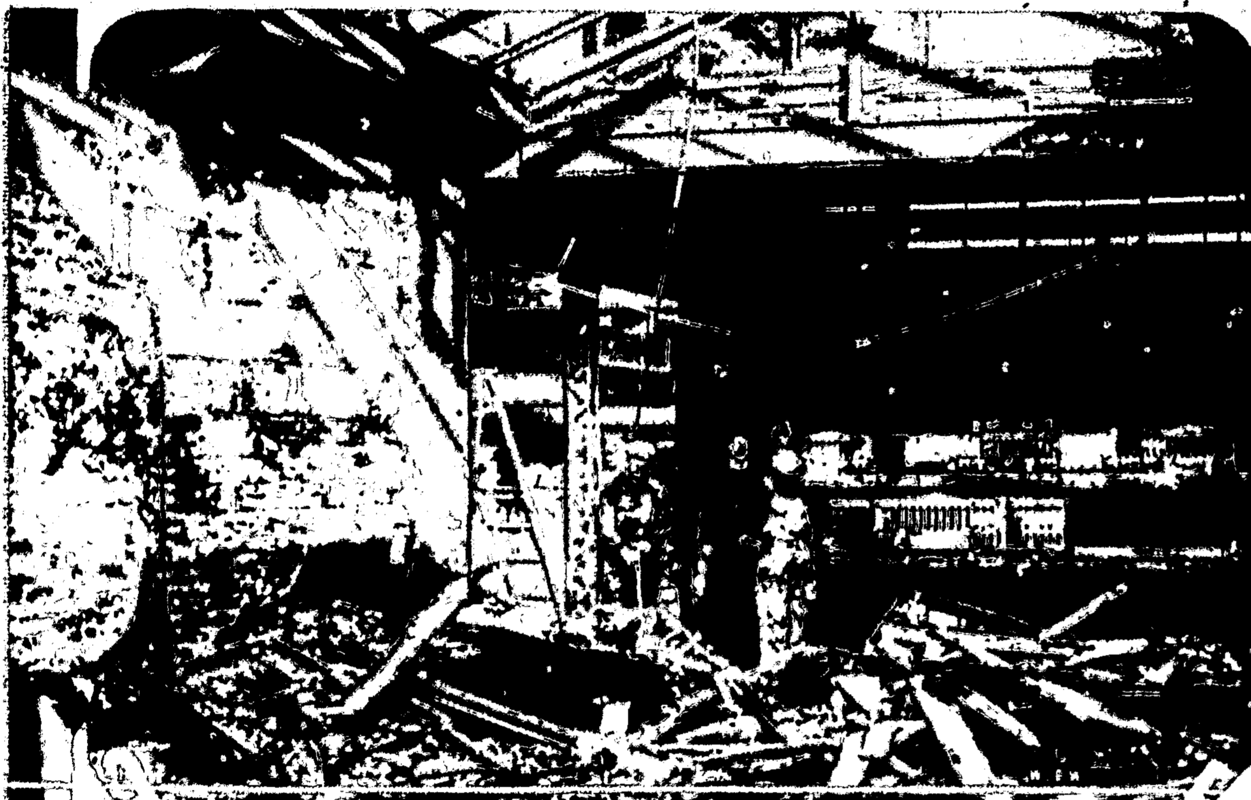
Valuable art works, including the model of the Capitol, were badly damaged by the mysterious fire that broke out in the west wing of the building. The photograph shows workmen clearing up the debris.
