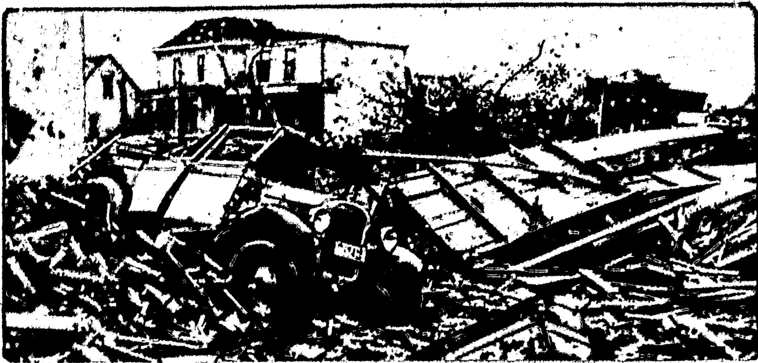
Tragic ruins which lie in the trail of destruction left by the series of giant twisters which tore through the east central portion of Minnesota and the west central portion of Wisconsin. Five persons were killed, 60 injured, thousands of dollars worth of property destroyed. The photograph was made at Randolph, Minn., one of the towns hardest hit.
