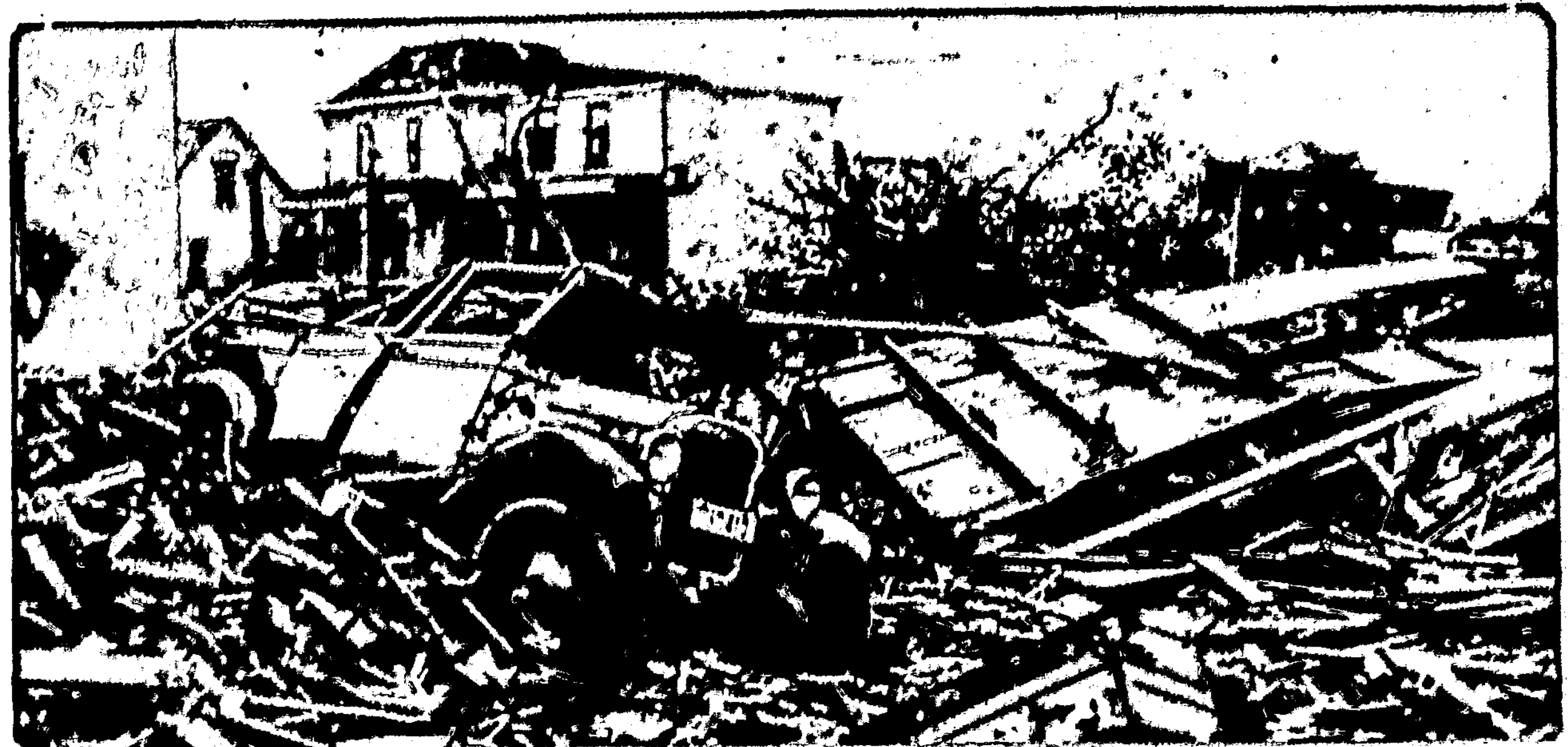
Tangle of ruins which lie in the trail of destruction left by a series of giant twisters which tore through the east central portion of Minnesota and the west central portion of Wisconsin. Five persons were killed, 60 injured, thousands of dollars worth of property destroyed. The photograph was made at Randolph, Minn., one of the towns hardest hit.
