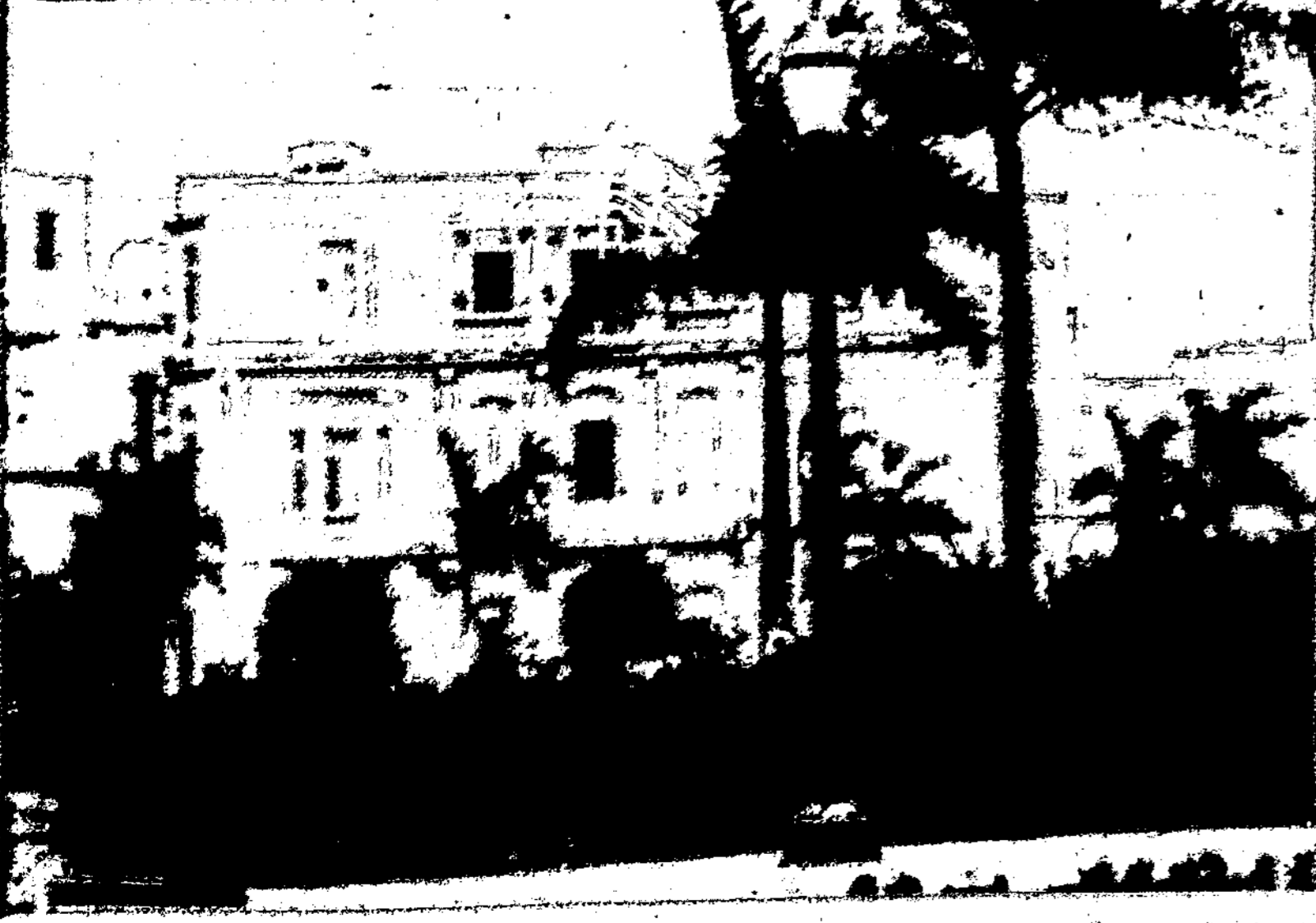
Standing proudly in the broad Avenida de la Misericordia, Havana's new "International Street," this structure now houses the United States embassy in Cuba, formerly quartered in a dark, cramped ancient section of the capital. The house is leased from the Marquesa de la Real Proclamacion, Spanish nobleman.
