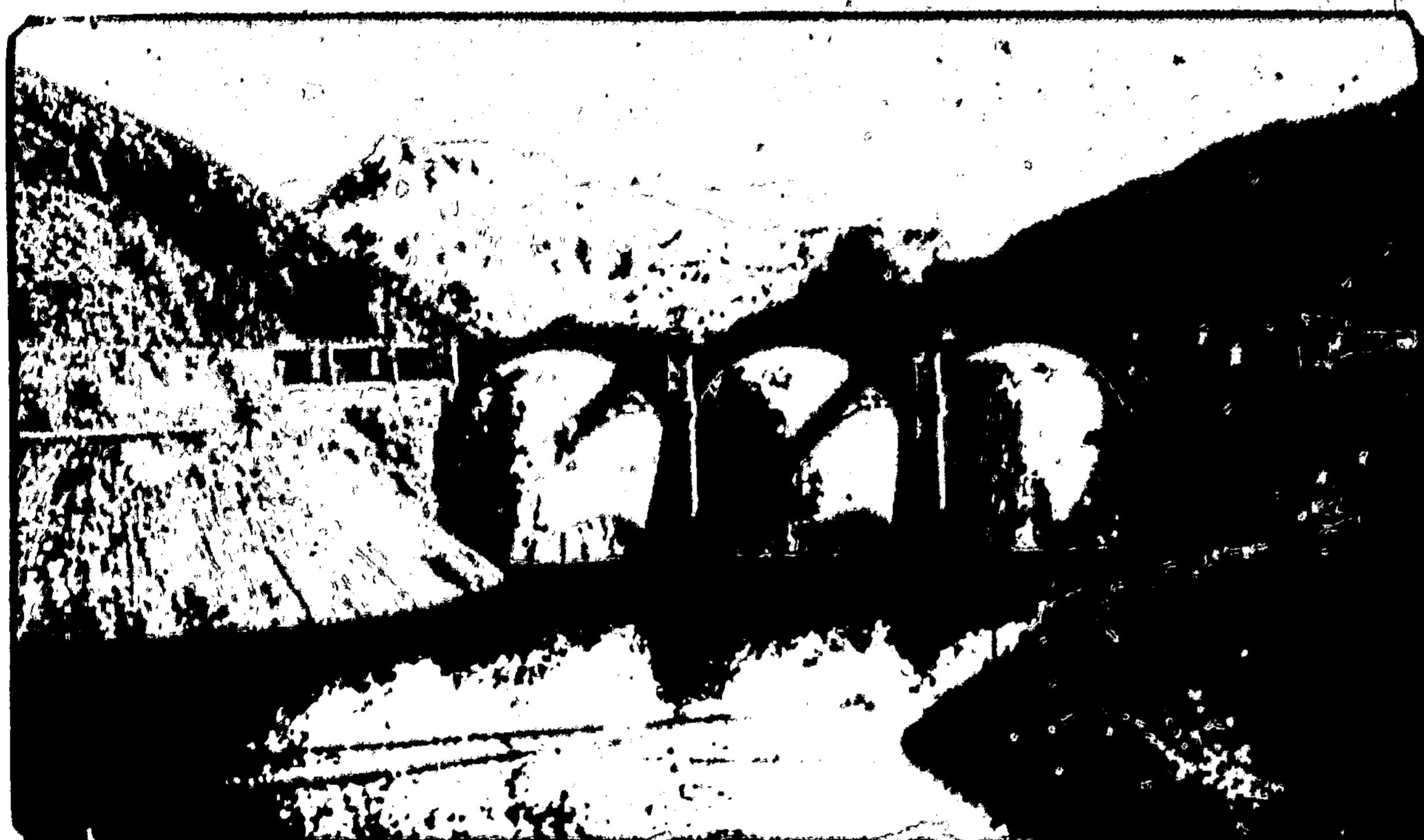
A new picture of the Coolidge dam in Arizona which reveals the impressiveness of the only multiple-domed dam in the world. It is situated about 135 miles southeast of Phoenix, and will serve to irrigate 100,000 acres of land along the Gila river.
