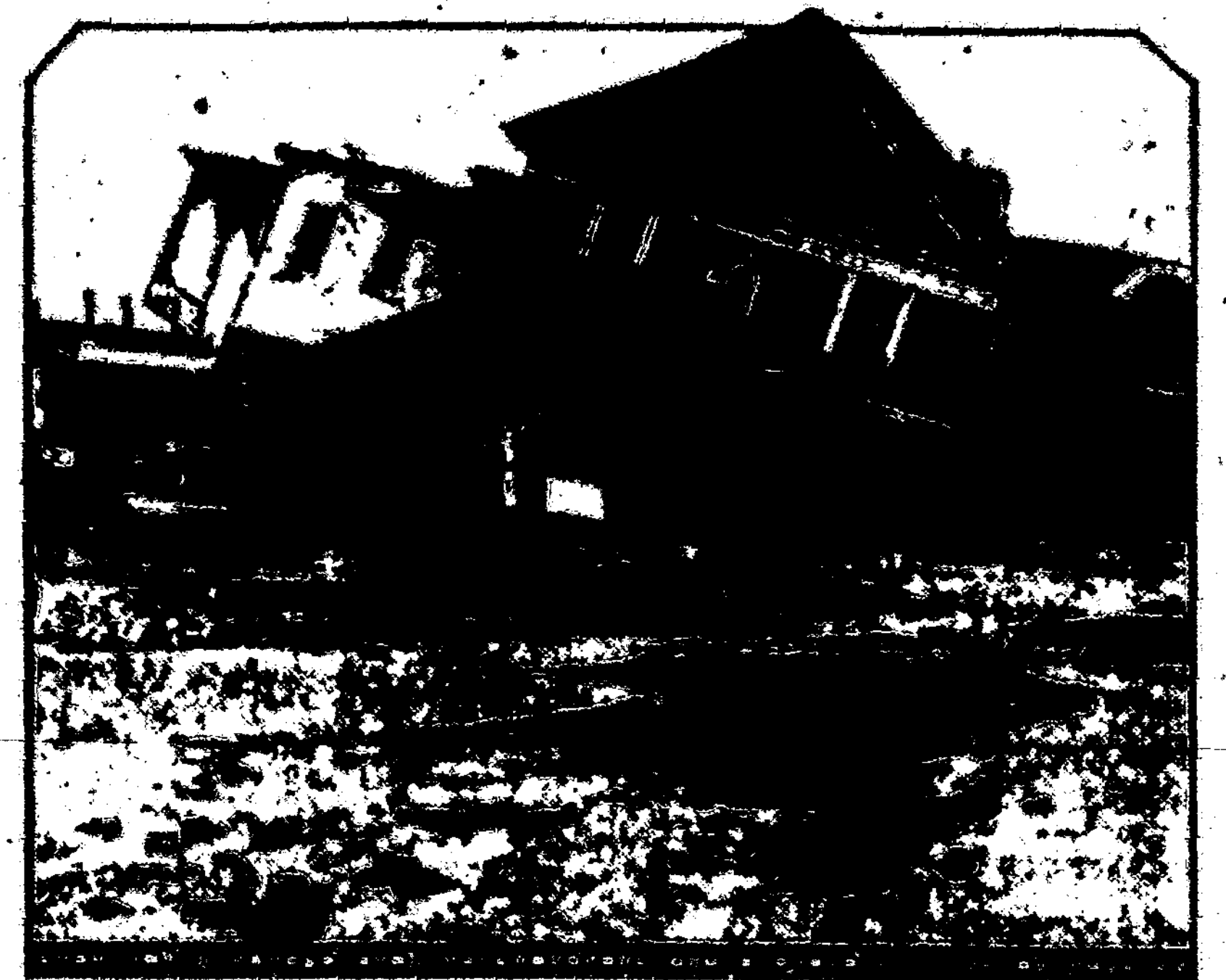
Wreckage of the Hinkman house, in Seabright, N. J., after it was demolished by the terrific gale which swept along the Atlantic seaboard. The heavy surf driven by the high winds washed away shore foundations at many resorts. Mountainous waves tore boardwalks to pieces and scores of homes were blown from their bases.
