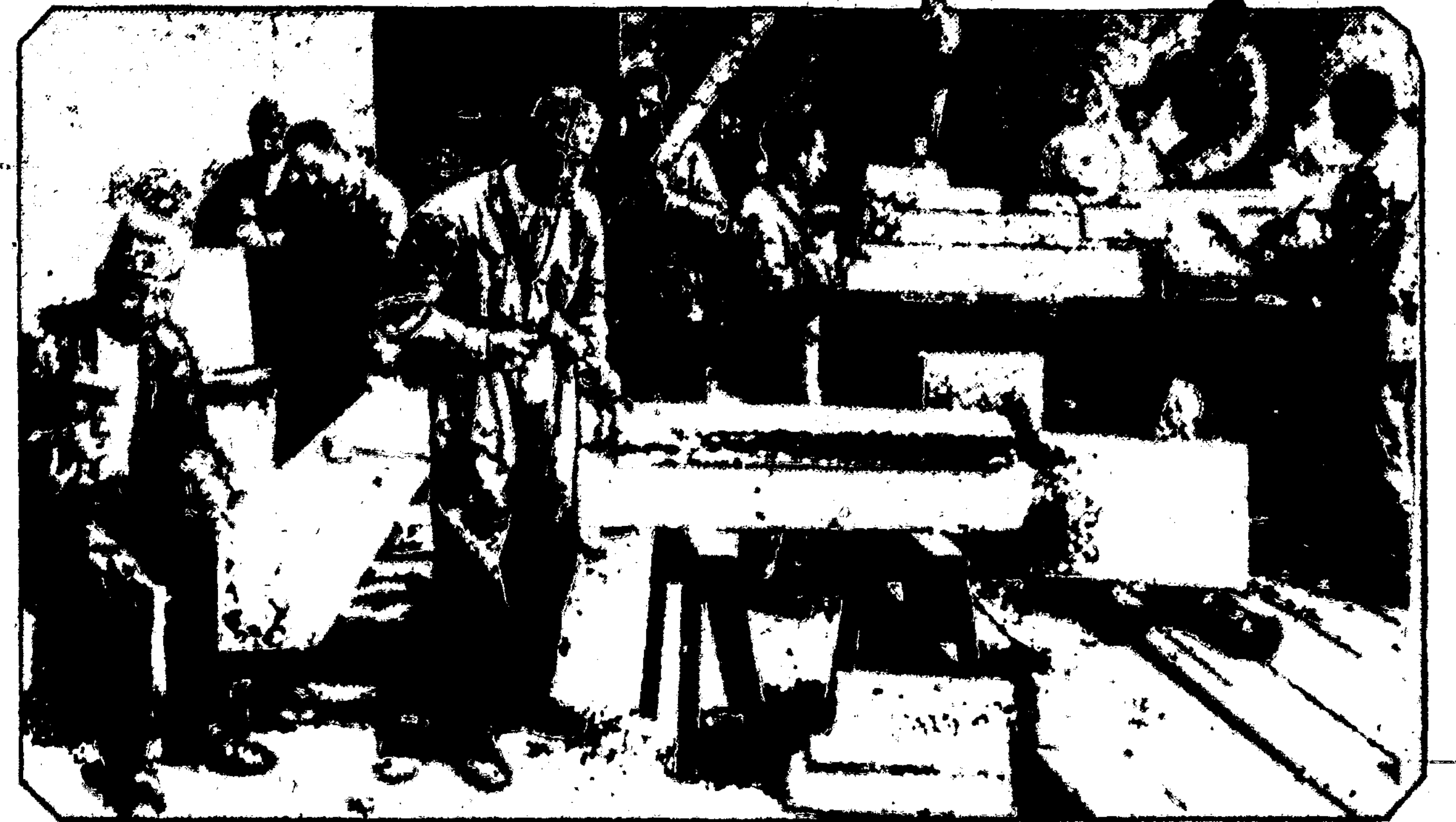
Workmen busy in the Vatican grounds cutting and trimming the marble for the restoration of the dome of St. Peter's cathedral, which has taken on more speed at the express wish of His Holiness.
