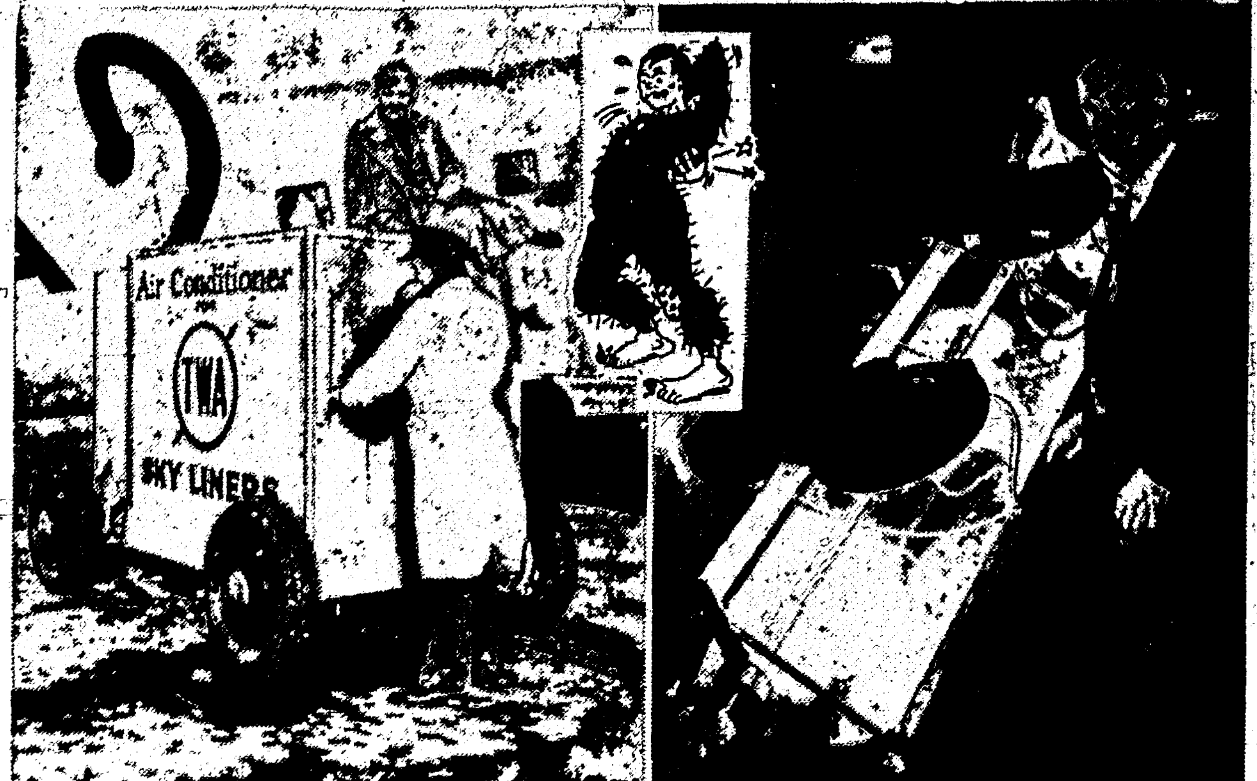
Keeping warm in winter has its problems for the poor fellow in the cartoon, who, like 12,000 other Americans, wears red flannels in the winter. The airlines have their warmth problem licked, for the same machine unit (left) which pumps cold air into the planes in summer fills them with warm air in winter; after they take off, a steam heating unit goes into operation. Some scientists predict that one day most of our heat will come from the sun via the solar machine, such as Dr. C. G. Abbot, of the Smithsonian Institution, is demonstrating (right).
