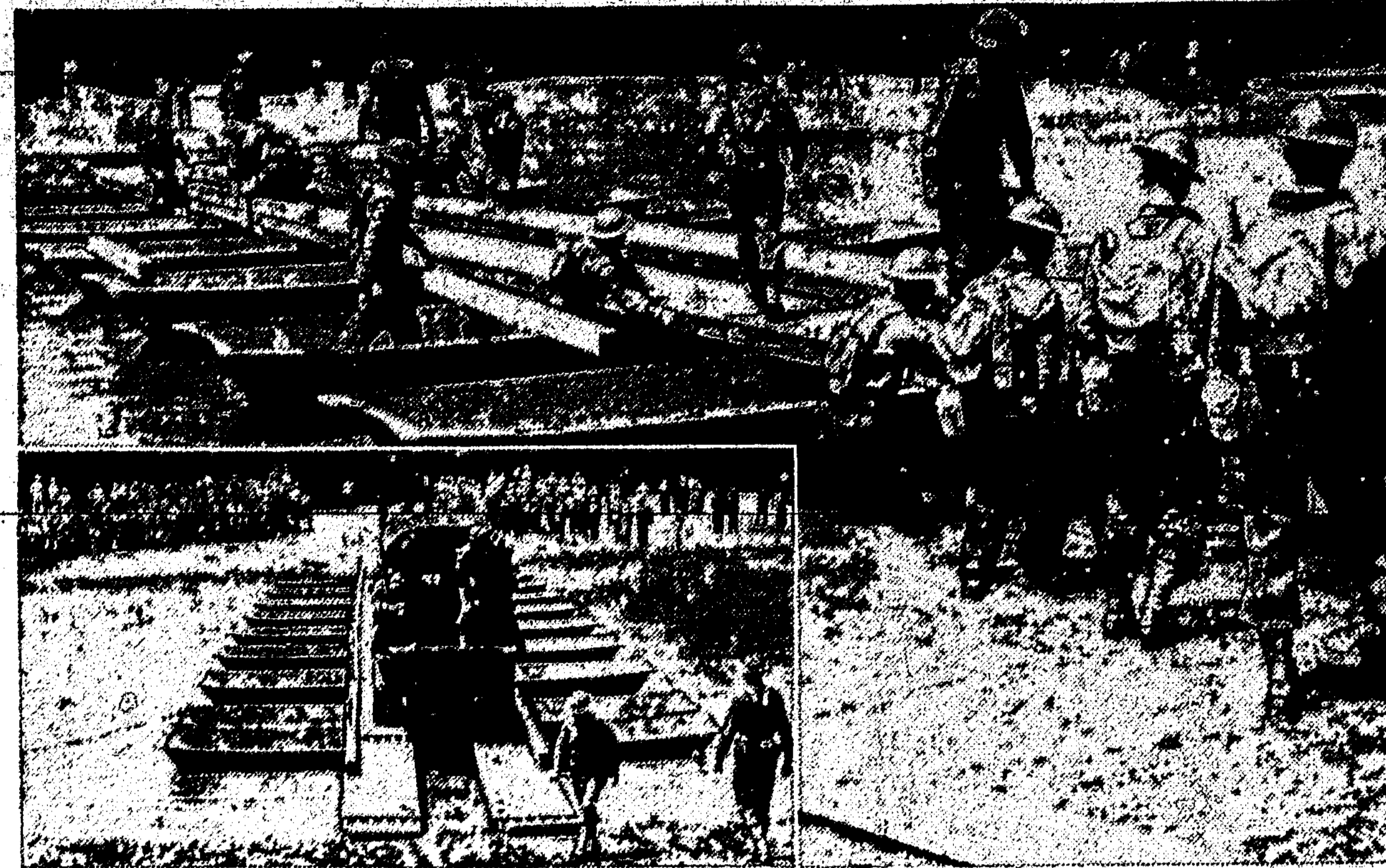
In a demonstration at Ft. Belvoir, Va., a motorized war-strength company of the Fifth Engineers dismantled from its trucks, unloaded equipment, and within 16 minutes constructed a 200-foot pontoon bridge strong enough to carry ammunition trucks. In picture at right, runways are laid across gunnels of light pontoons. Inset: Company "E" of the Fifth Engineers is shown crossing waterway on bridge.
