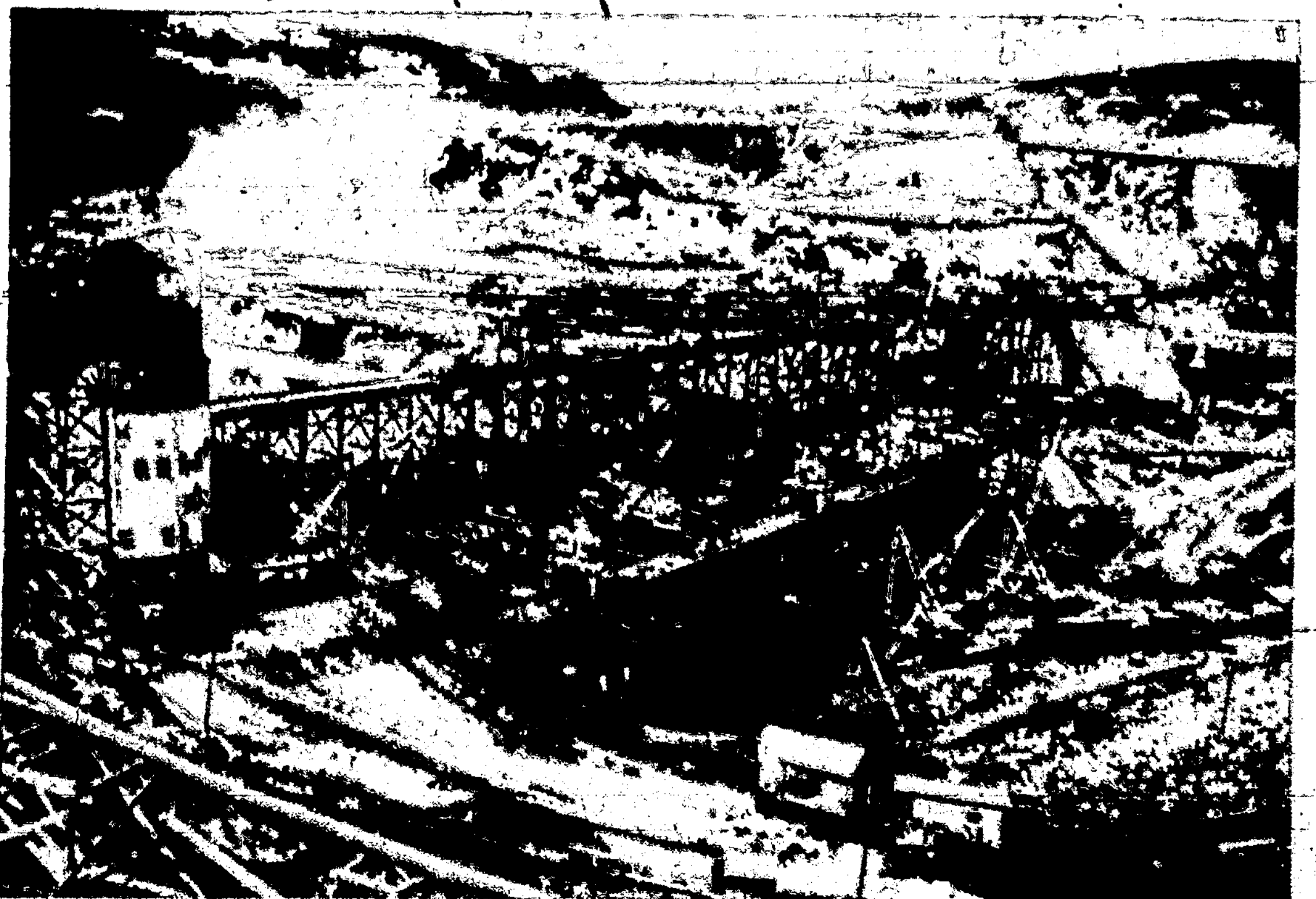
Work is being speeded on the Grand Coulee dam on the Columbia river in the state of Washington, which will eventually cost more than $113,000,000. The giant concrete mixer at left and the second on the opposite side of the river deliver concrete to cars which operate on a trestle.
