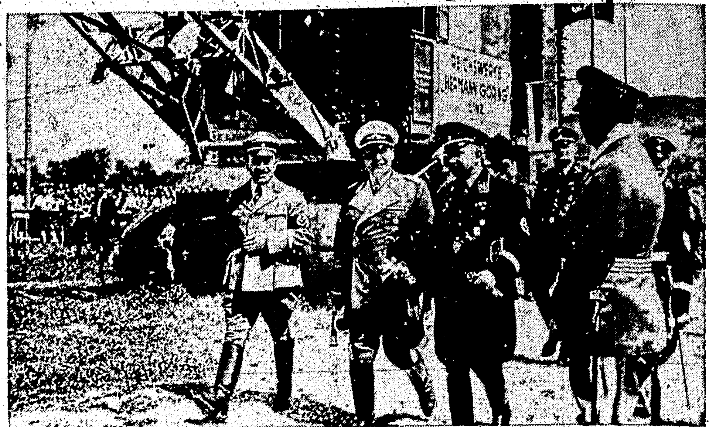
Field Marshal Hermann Goering (center) inspecting the site of the new Hermann Goering iron foundries at Linz, Austria, after laying the cornerstone recently. In his dedicatory speech he said, "Let others have gold, we are happy to have iron."
