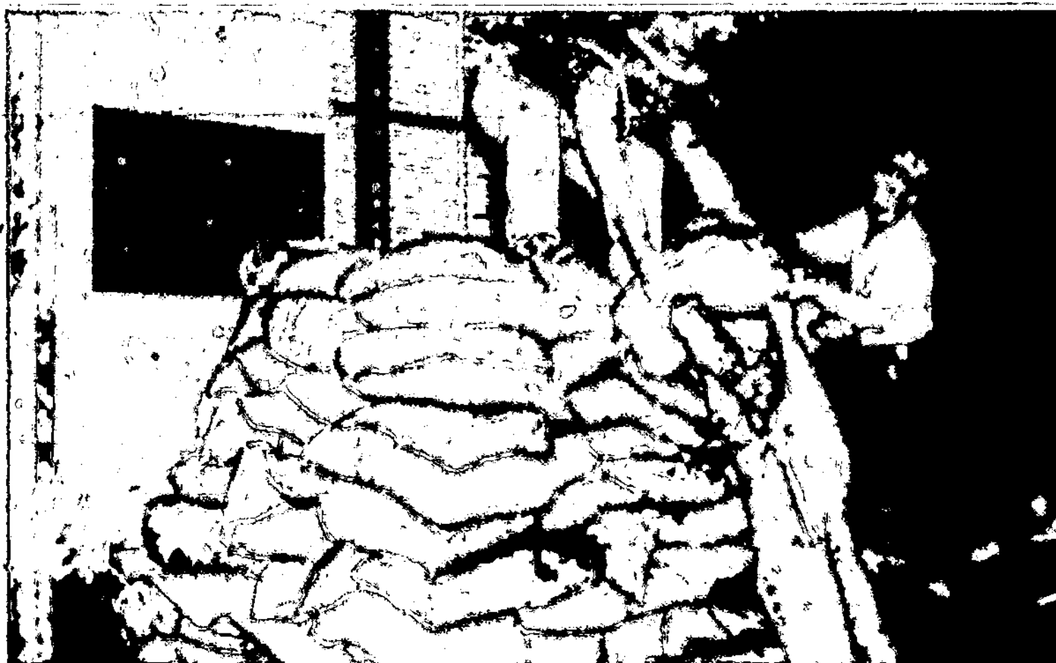
Following almost nightly air raid alarms and blackouts of San Francisco since the start of the war, the Pacific Telephone and Telegraph company has installed a sandbag barricade across the front of their building. Workmen are shown here erecting the wall of sandbags, which will protect vital telephone equipment from possible enemy bombs.
