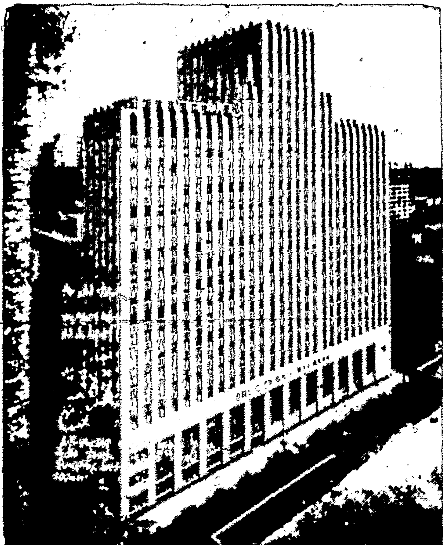
First skyscraper to be completed since the war is that of the City National Bank in Houston, Texas, a 24 story structure of steel, concrete, brick and stone. Structural steel for the building, amounting to 3,378 tons, was provided by United States Steel Corporation.
