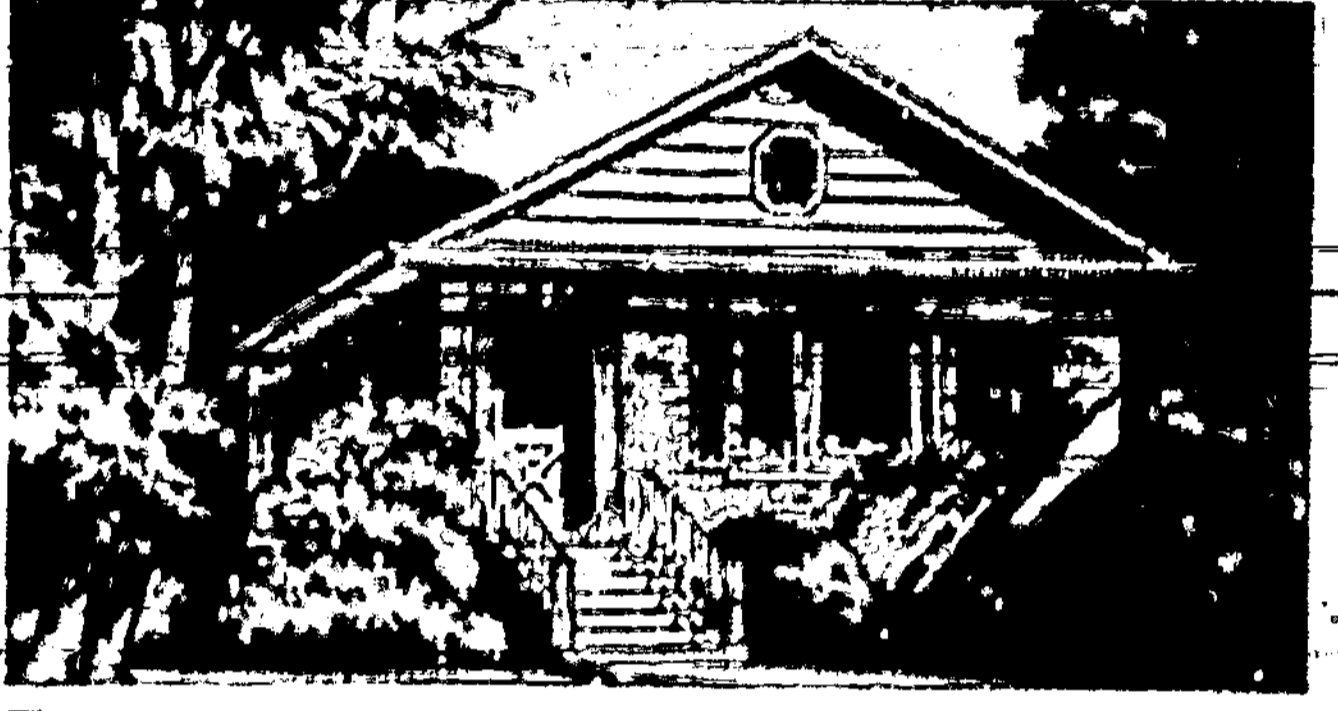
The door is moved to the front, entrance brick work replaced.
