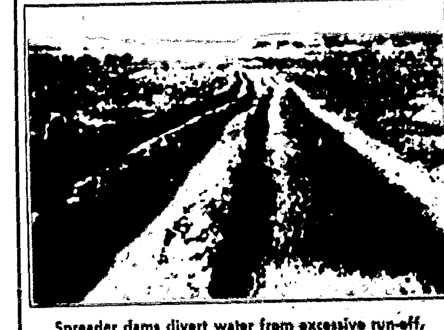
Spreader dams divert water from excessive run-off, checking erosion in active gullies
