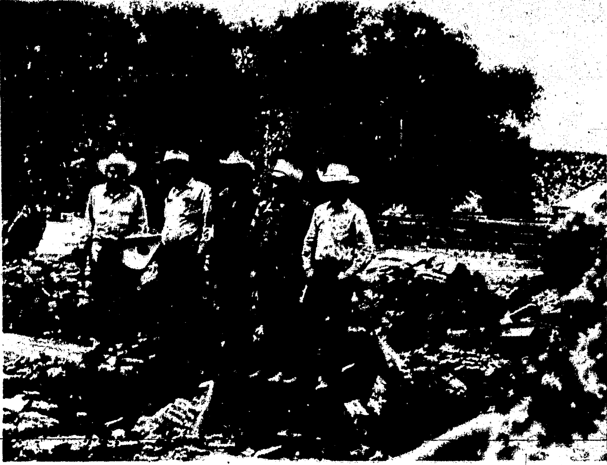
VIEWING THE WRECKAGE — Charley Jones, one of the Smokey Bear Stampede rammers on the left, Leroy McKnight and crew are looking over the remains of the old school on fair grounds at Capitan. The walls were being pushed in Monday to clear the way for the Stampede this weekend.
