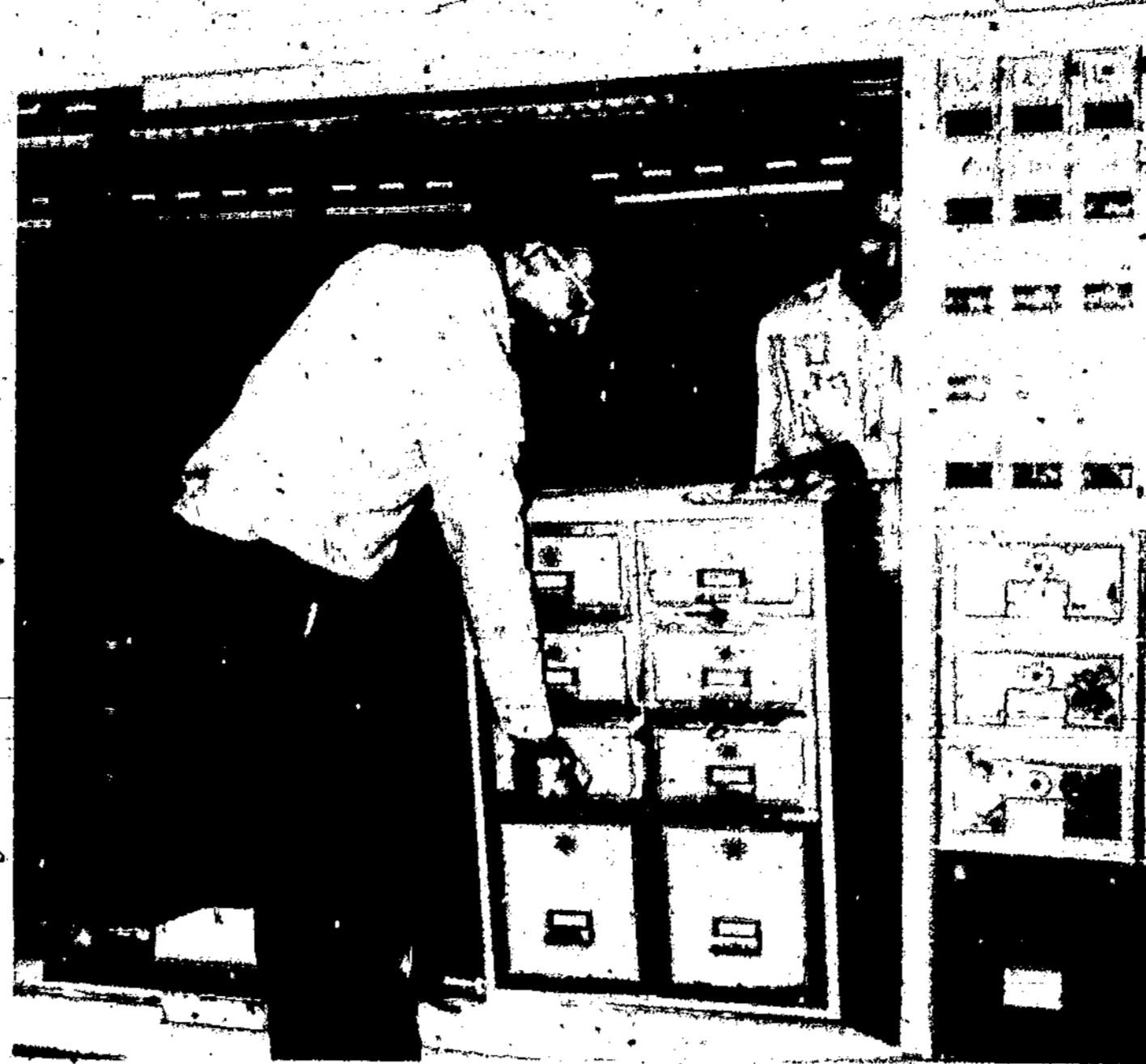
MAIL BOXES GOING IN — It took a lot of carpentry work to shape up the new Carrizozo postoffice to such a fine building. Glad we got to help — Leandro Jr. and Henry Vega.
