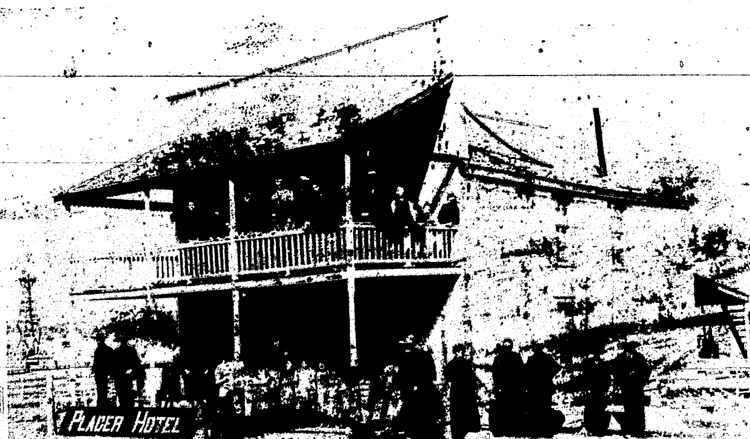
PLACER HOTEL IN NOGAL ABOUT 1885 -- At the time the Helen Rae and Parsons mines were in full production the town of Nogal was a going place with two newspapers, several saloons, livery stables and general merchandise stores. The boom
