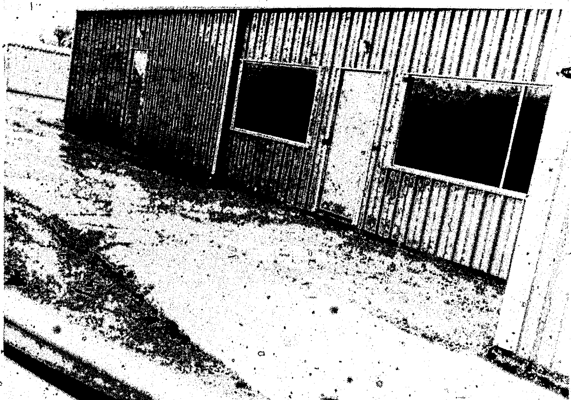
Town of Carrizozo has not had a real heavy rain so far this year but there has been sufficient runoff by new town hall to make shallow lake in
