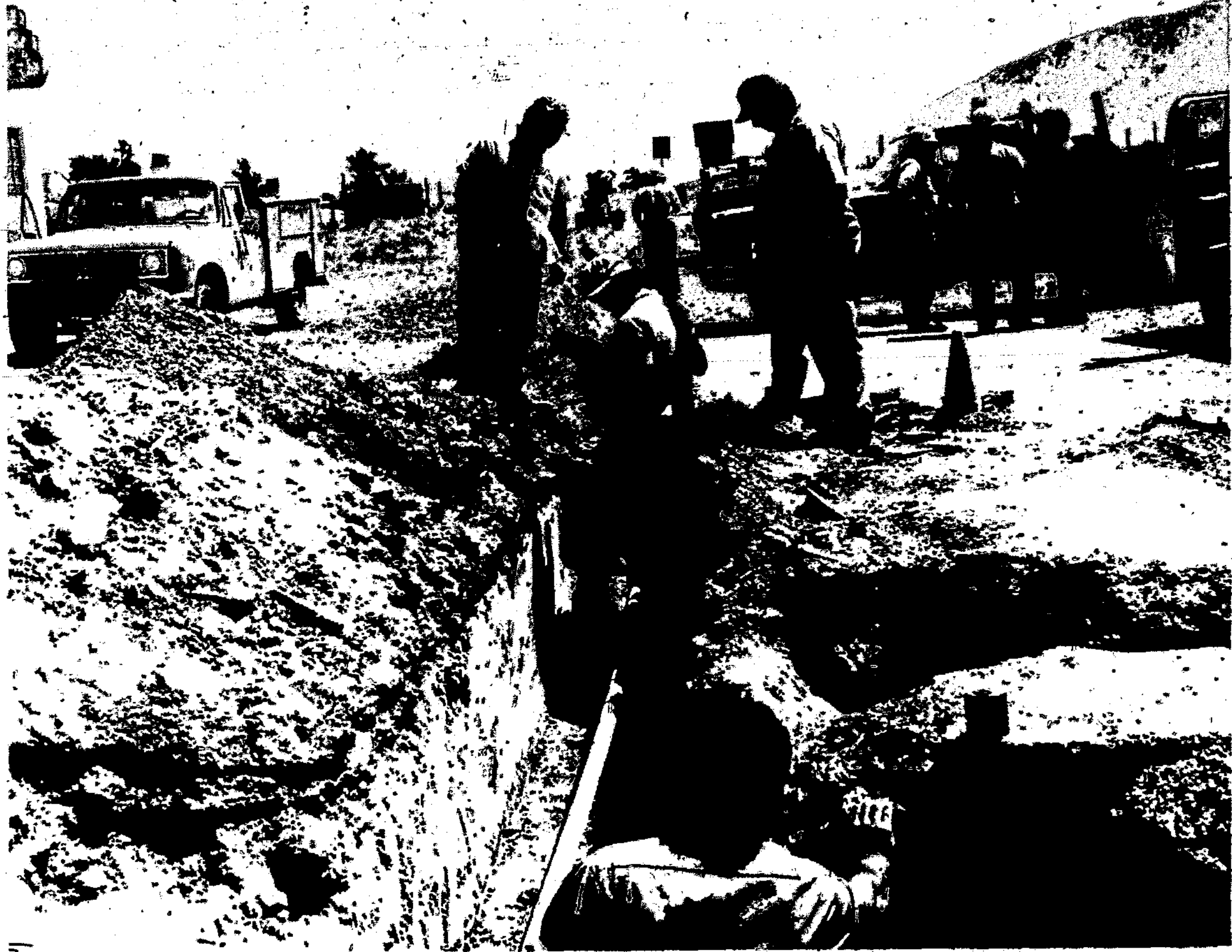
Joe Vega, foreman, District 2 Patrol, Carrizozo, State Highway Department was supervising Tuesday and Wednesday the laying of a water line from Carrizozo to the patrol headquarters out U.S. 54 toward Corona. A well at the patrol headquarters produces "bad" water; thus the mile-long new water line to obtain Carrizozo city water.
