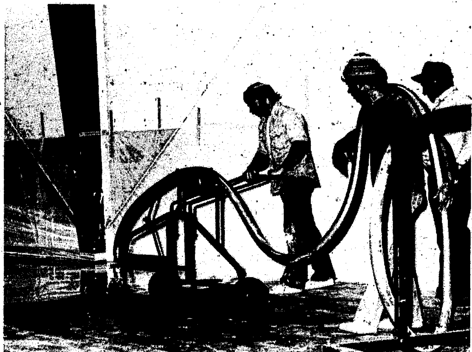
The new bright yellow Carrizozo gym floor was poured last week. Yes, POURED! Instead of hardwood, specialists now use polyurethane for sports floors of all kinds, even outside tracks. The "Robbins Proturf" will be 3/4 inches thick
