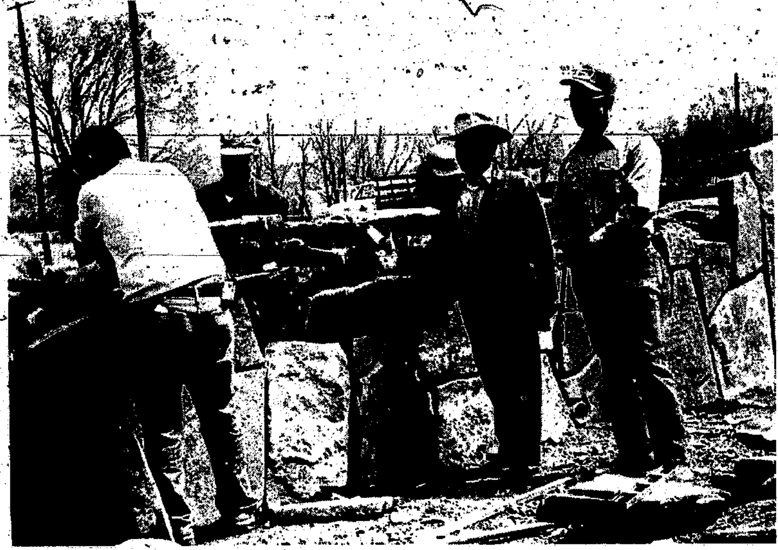
First stage construction of the grounds at the Smokey Bear State Park in Capitan includes a rock wall. Parks department physical plant manager Joe Rodriguez and Mayor Jay Johnson
