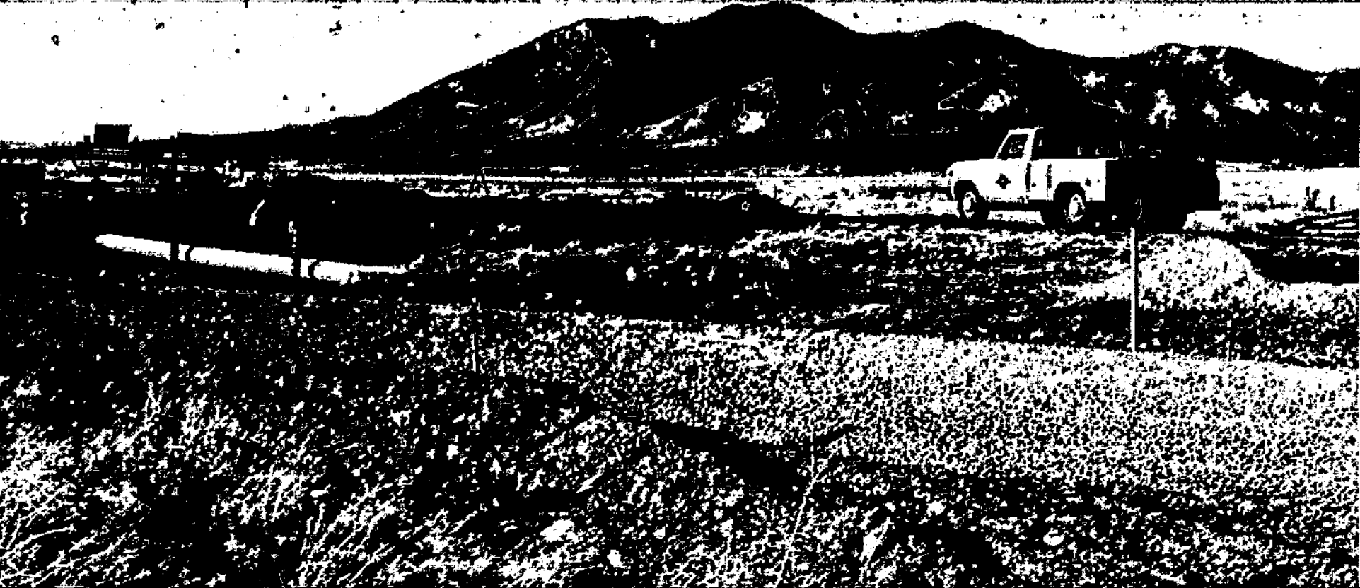
Bridge construction has started 1 1/2 mile east of the Hiway 380, Hiway 37 intersection. The bridge is being
