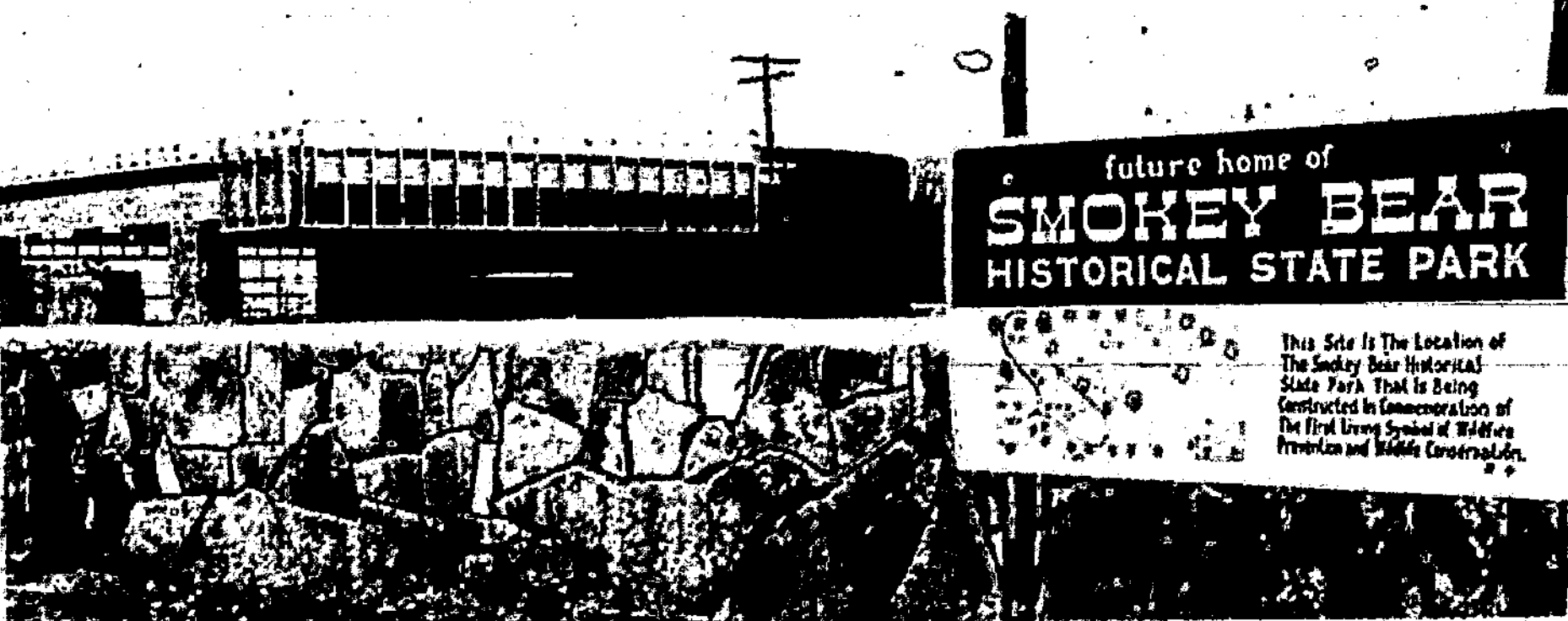
File photo while under construction-full story on opening next week-
