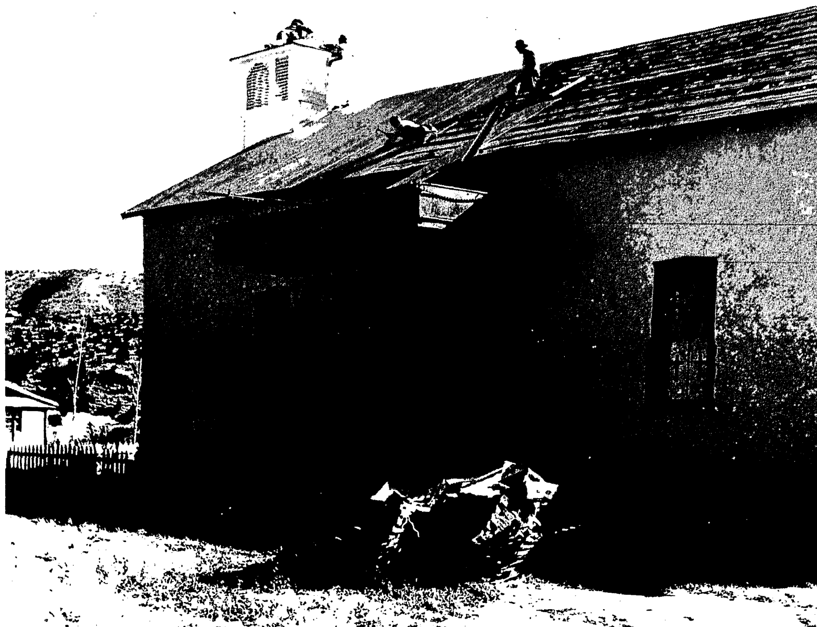
WORKERS reroof San Juan Church at Lincoln State Monument as part of a restoration project.
