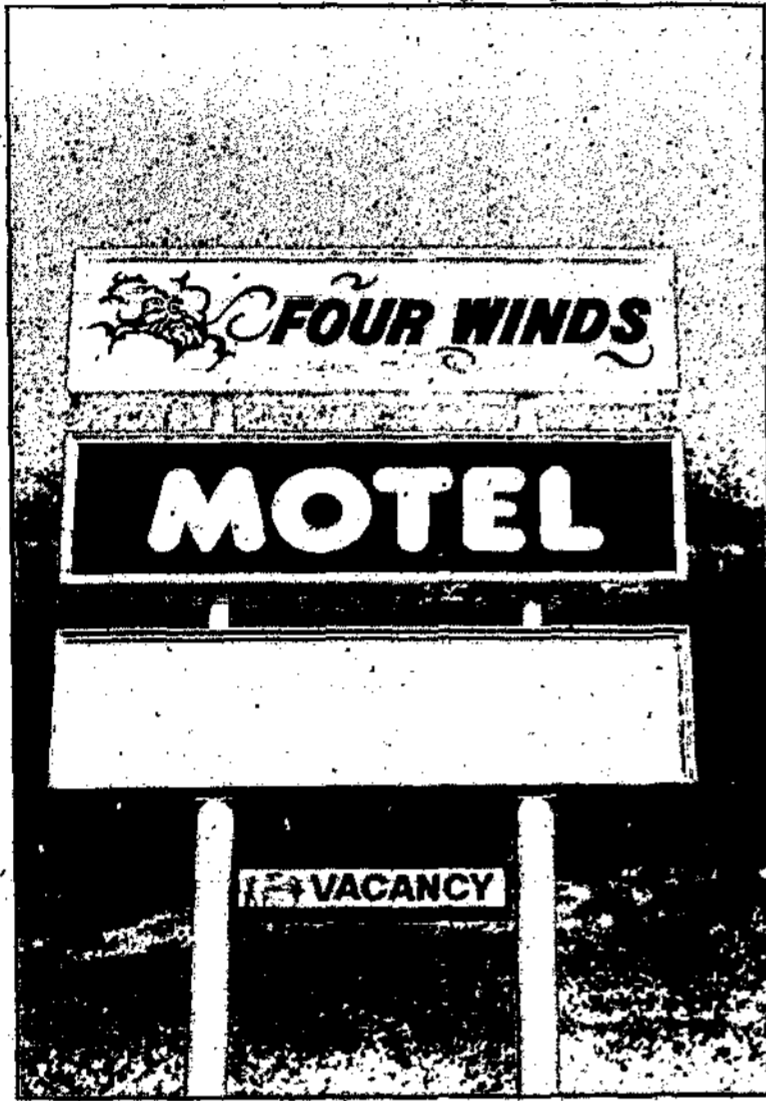
SIGN UP—Willie Silva's new Four Winds Motel sign goes into place. Ken Wells, contractor, says the construction is on schedule and that the new motel will be open Oct. 1.
