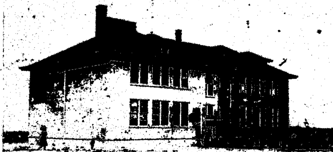
Original Carrizozo Public Schools building as it looked in 30's... later remodeled in late 50's and finally torn down in '65 after having served its usefulness. (Photo courtesy of J.S. Stearns)
