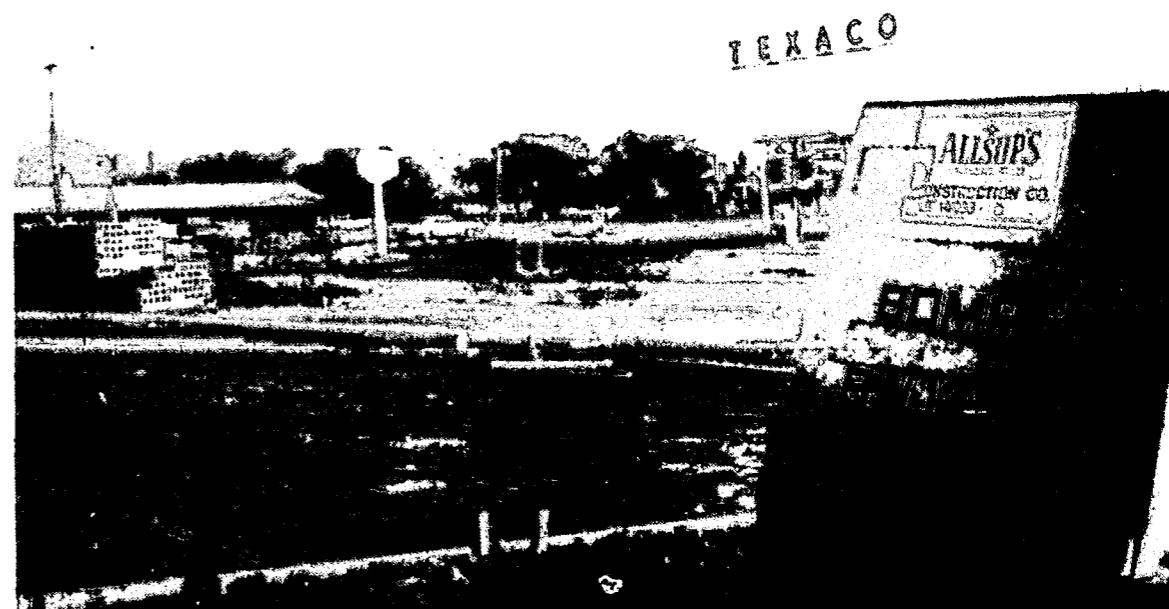
WORKMEN have completed most of the groundwork for the new Allsup convenience store in Carrizozo. The store is located at the intersection of Highways 54 and 380. The building is expected to be completed in another month.
