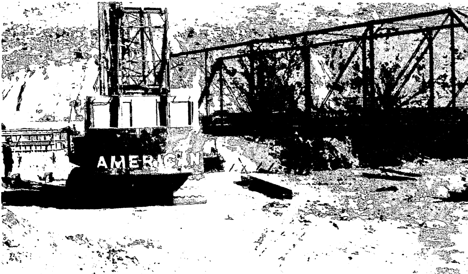
THIS OLD bridge, located one mile west of Picacho, is being replaced by a new one. The old bridge will continue to stand as a state landmark. Originally built in 1909 over the Pecos River east of Roswell, it was moved to its present location in 1941. Hasse Contracting Company of Albuquerque expects to have the job done by the end of February. Asphalt will be laid when the weather permits.
