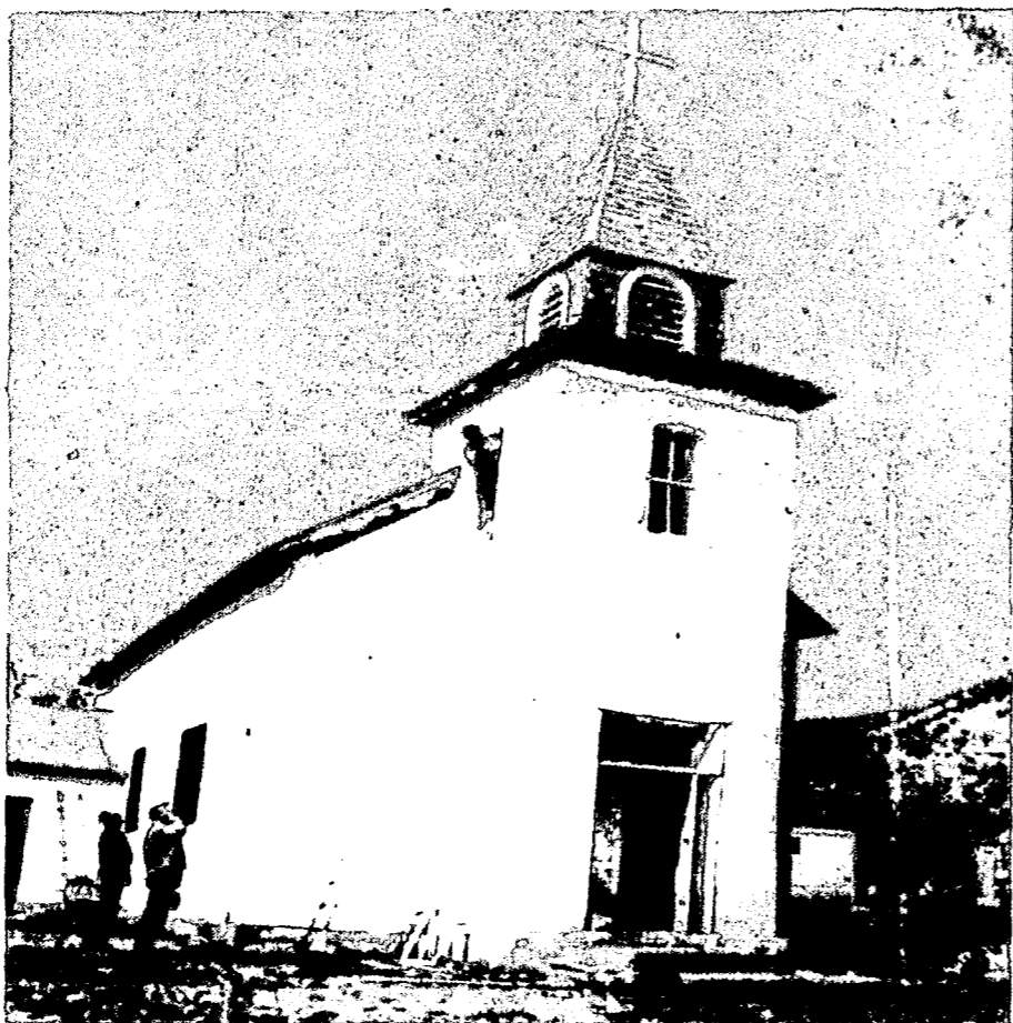
THE OLD SAN PATRICIO CHURCH is in for restoration. Some of those doing the work are Joe Gutierrez and John Hamilton, on the ground, and Rufino Herrera, on the ladder.
