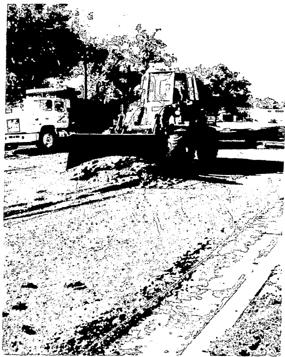
REPAVING WORK begins on E. Ave. in Carrizozo. Late last week, crews ground up the old pavement from 8th St. to Central Ave. By Wednesday, crews were removing the ground up materials, readying the roadway for the paving. The repaving project is being financed by a New Mexico House Memorial through the New Mexico State Highway and Transportation Dept.
