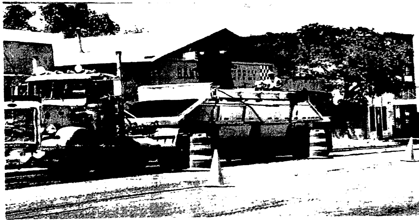
CONSTRUCTION OF HIGHWAY 54 ON CENTRAL AVE. IN CARRIZOZO continues this week as C.S. McCrossan, Inc. crews work. Milling of the roadway on the .9 mile project is almost completed and paving should begin next week. Motorists are asked to not park on Central Ave. in the construction zone until after the project is completed. Everyone agrees the inconvenience will be worth it when Highway 54 through Carrizozo is completed.
