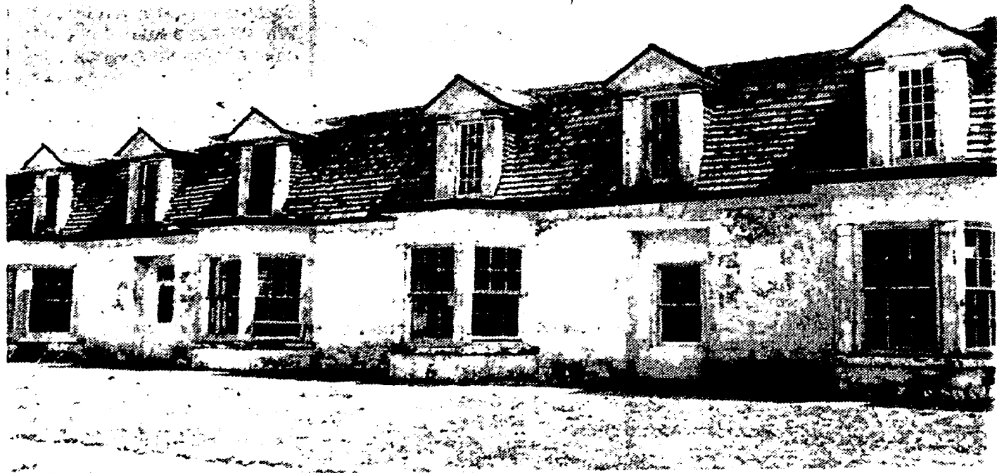
SAVED BY A NEW ROOF. One of the oldest buildings at Fort Stanton recently received a roof of new cedar shake shingles, thus preserving the old structure for a few more years. However there is no access to the building, which is not being used at this time. The project was planned before the women corrections facility moved into Fort Stanton, said Warden Sandra McFadin.
