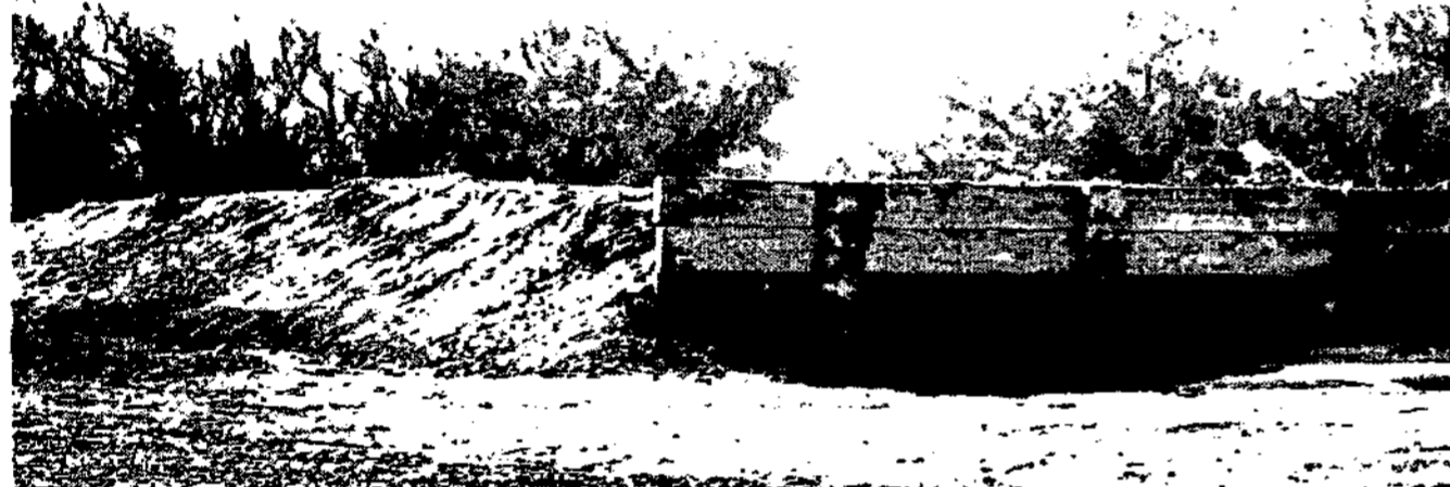
TRASHY RAMP. Lincoln County Solid Waste Authority with help from the town of Carrizozo recently constructed this ramp so trash collection trucks can dump into a walking floor trailer that will be hauled directly to the regional landfill south of Alamogordo. The ramp is located north of Evergreen Cemetery on town land. LCSWA hopes the ramp and transfer location will cut hauling costs.
