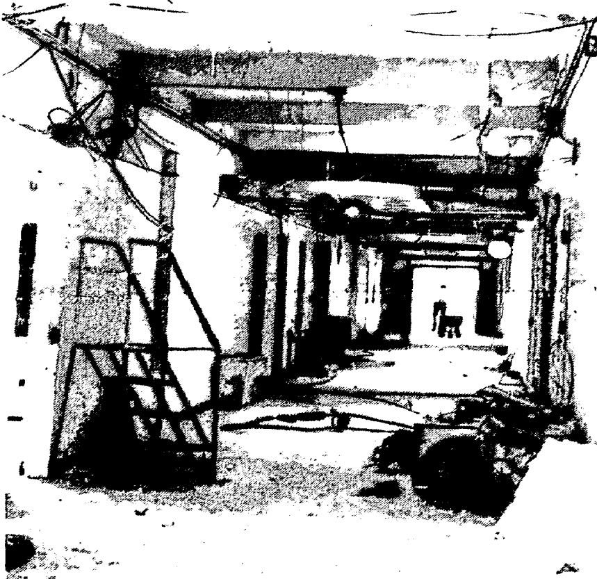
HARD HAT AREA. Carrizozo Elementary School is now a hard hat area, thanks to a remodeling project financed with state critical capital outlay funds which are derived from lottery proceeds. Workers with Rebcon Services, Inc. construction company of Albuquerque are now in the demolition stage, tearing out old ceilings, old wiring and duct work, and getting ready to knock out the north walls to extend the north side classrooms by 10 feet. The project will also involve remodeling of the middle school area to provide ADA handicapped accessible toilets and a new science room area. Remodeling is expected to be totally completed by October 31. Project supervisor is Frank Sierra.
