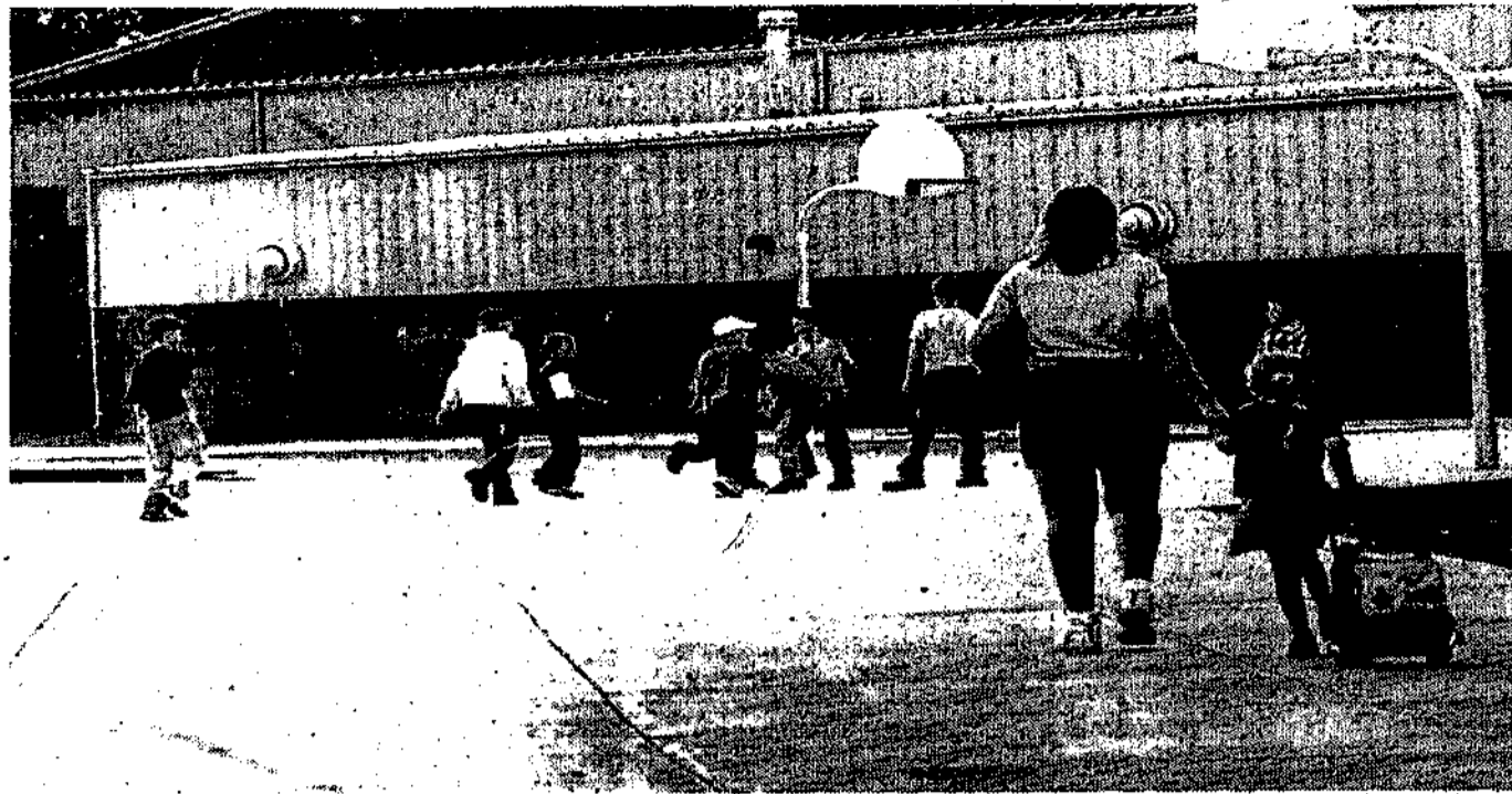
NEW PLAY AREA attracts students waiting for class on the Capitán school campus. New landscaping and play areas and classroom additions were constructed with bond funds. The new improvements were showcased during an open house and back to school night picnic and watermelon feed, sponsored by the Capitán PTA on Tuesday. The event was well attended.
