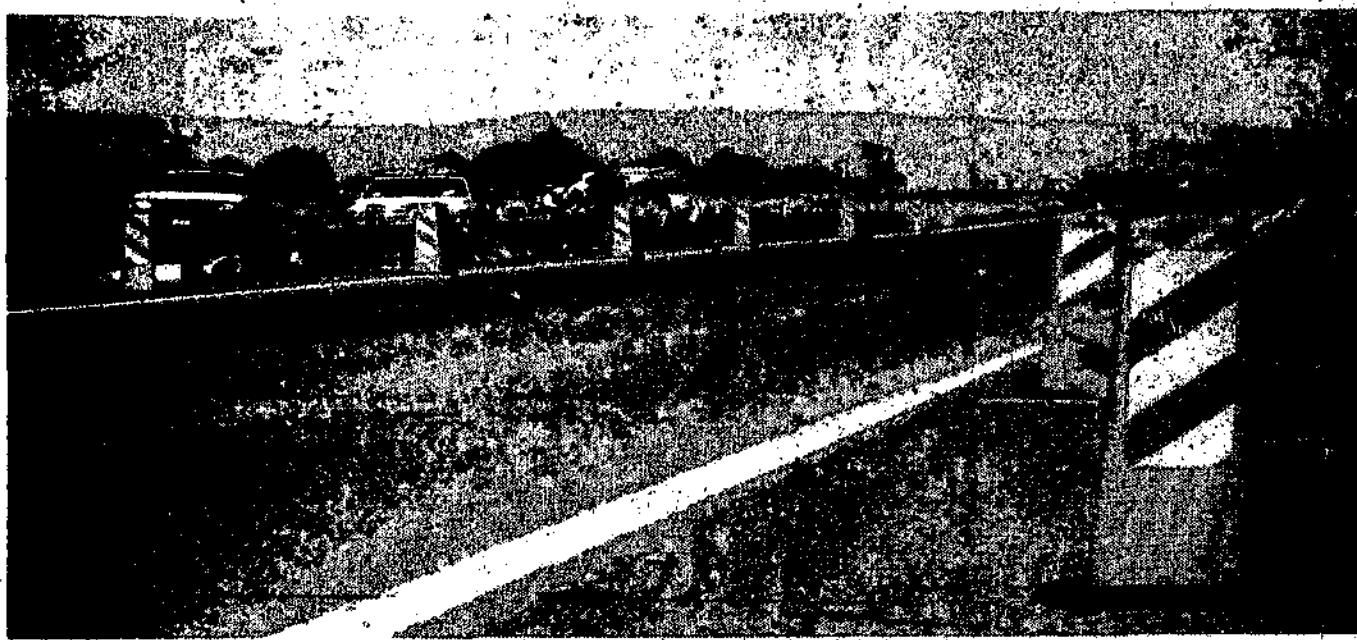
SLOW DOWN. Motorists on Highway 380 just east of Carrizozo need to slow down for reduced speed zones to 35 miles per hour in construction work zones. Hamilton Construction crews are breaking out concrete bridge components to allow for widening of the roadbed. The project is scheduled to be completed by late summer.
