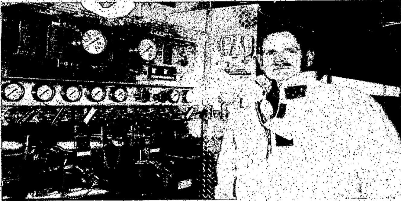
CARRIZOZO VOLUNTEER FIRE DEPARTMENT'S Training Officer, John Tate, is shown next to the control panel of the department's newest fire engine.
