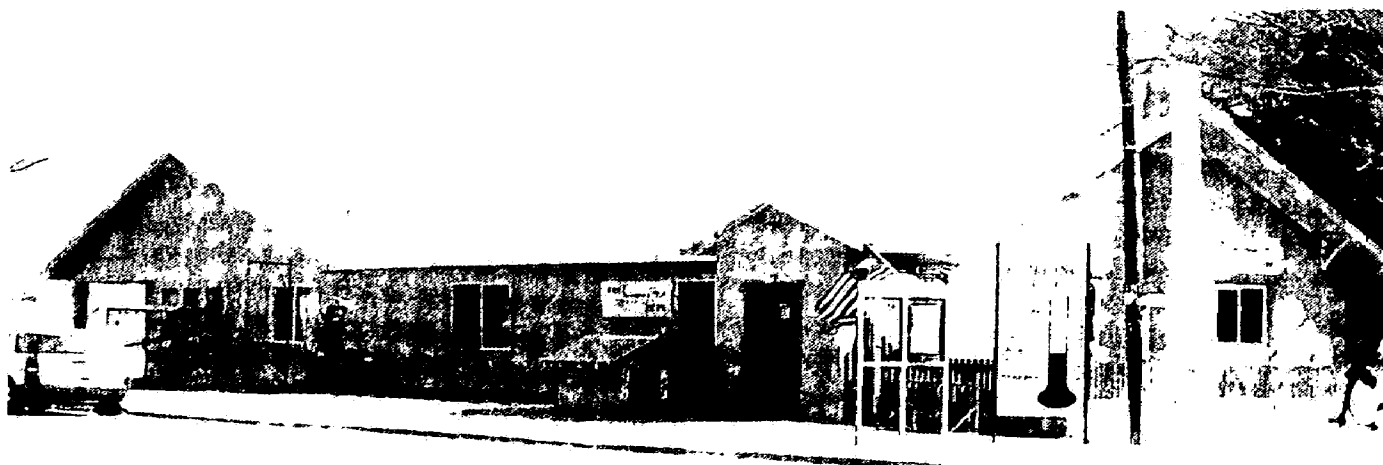
THE CAPITAN PUBLIC LIBRARY continues to serve area residents, and offers several programs for children and adults. The new addition to the library is nearing completion. The library will hold a fund-raiser plant and gift sale this Saturday, beginning at 8:00 a.m. and ending at 2:00 p.m. or until the plants are sold out.
