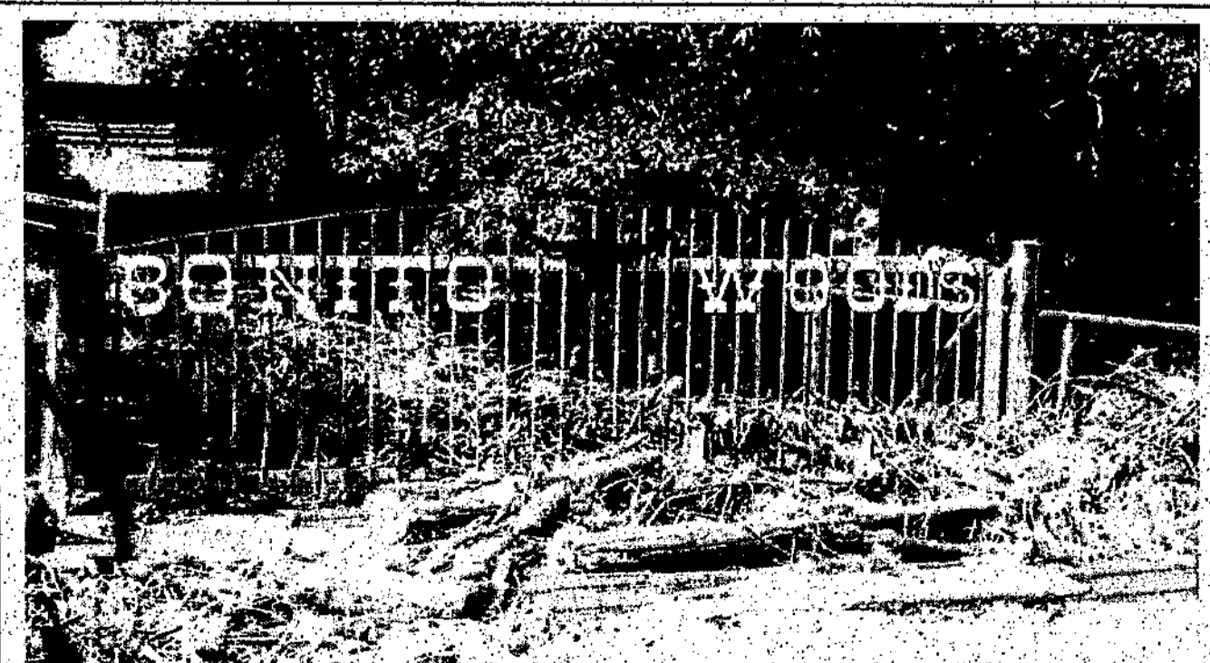
BONITO WOODS -- City and county crews and residents have been working hard in flood-damaged parts of the county to clean up in the aftermath of flooding that left hundreds of people stranded. As this photo illustrates, much is left of be done. (Photo courtesy of Tim Brazie)
