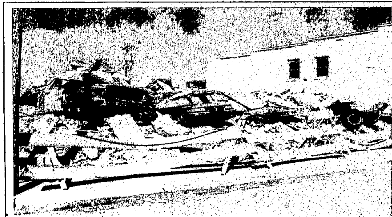
ONE MAN'S TRASH is another man's treasure, and this pile of broken concrete and crushed cars is part of the beauty of movie magic as one block of 12th Street in Carrizozo continues to be transformed into a desolate post-apocalyptic scene. (Photo by Patrice Brazie)
