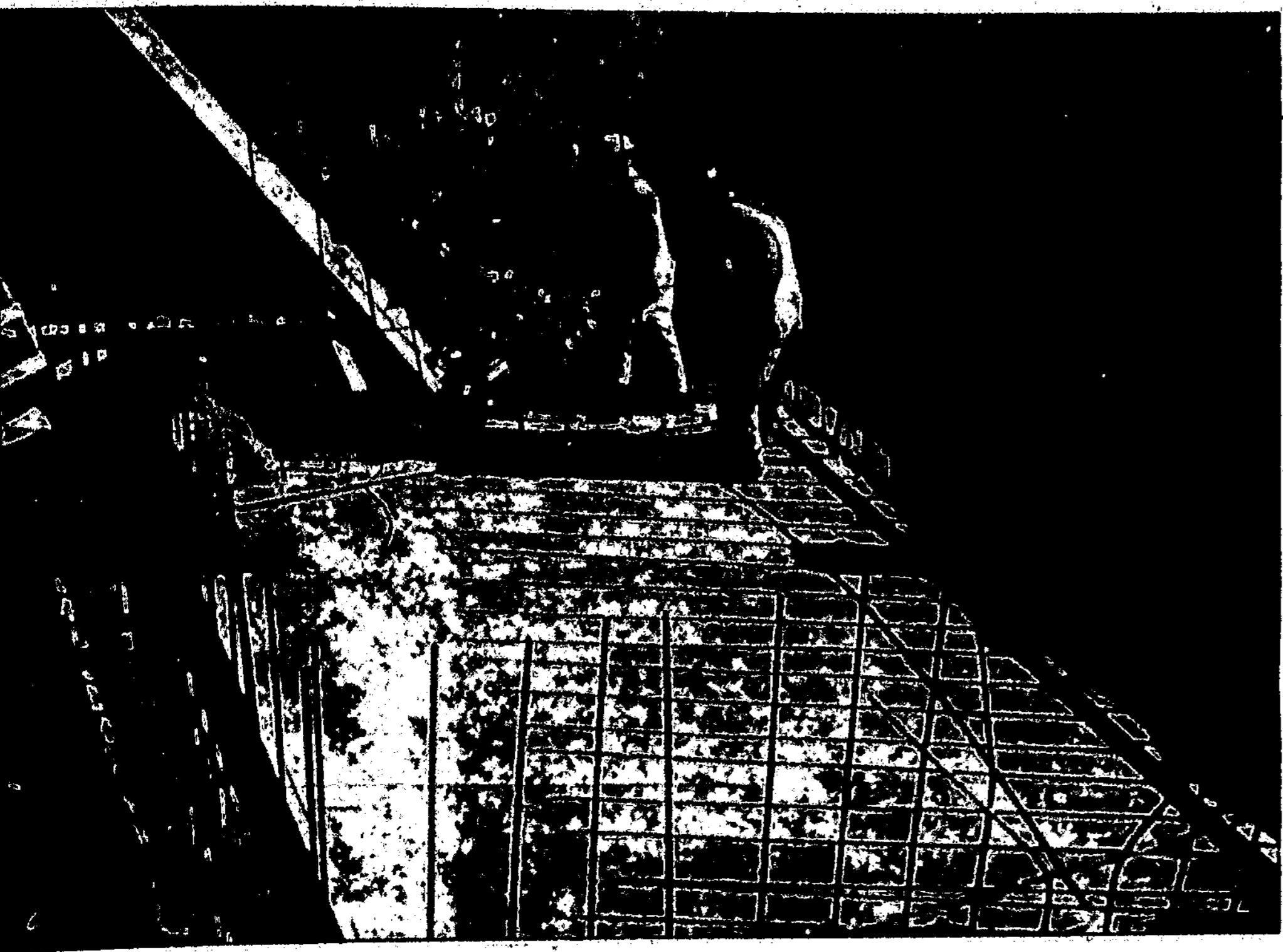
HUGE SEPTIC TANK —Construction is almost completed on huge septic tank in White Mountain Park to serve the sport shop, dining facilities and rental lodges Sierra Blanca Corporation is building there for a winter and summer resort. Other view shows crane being used to dig lateral lines for the sewer system.
