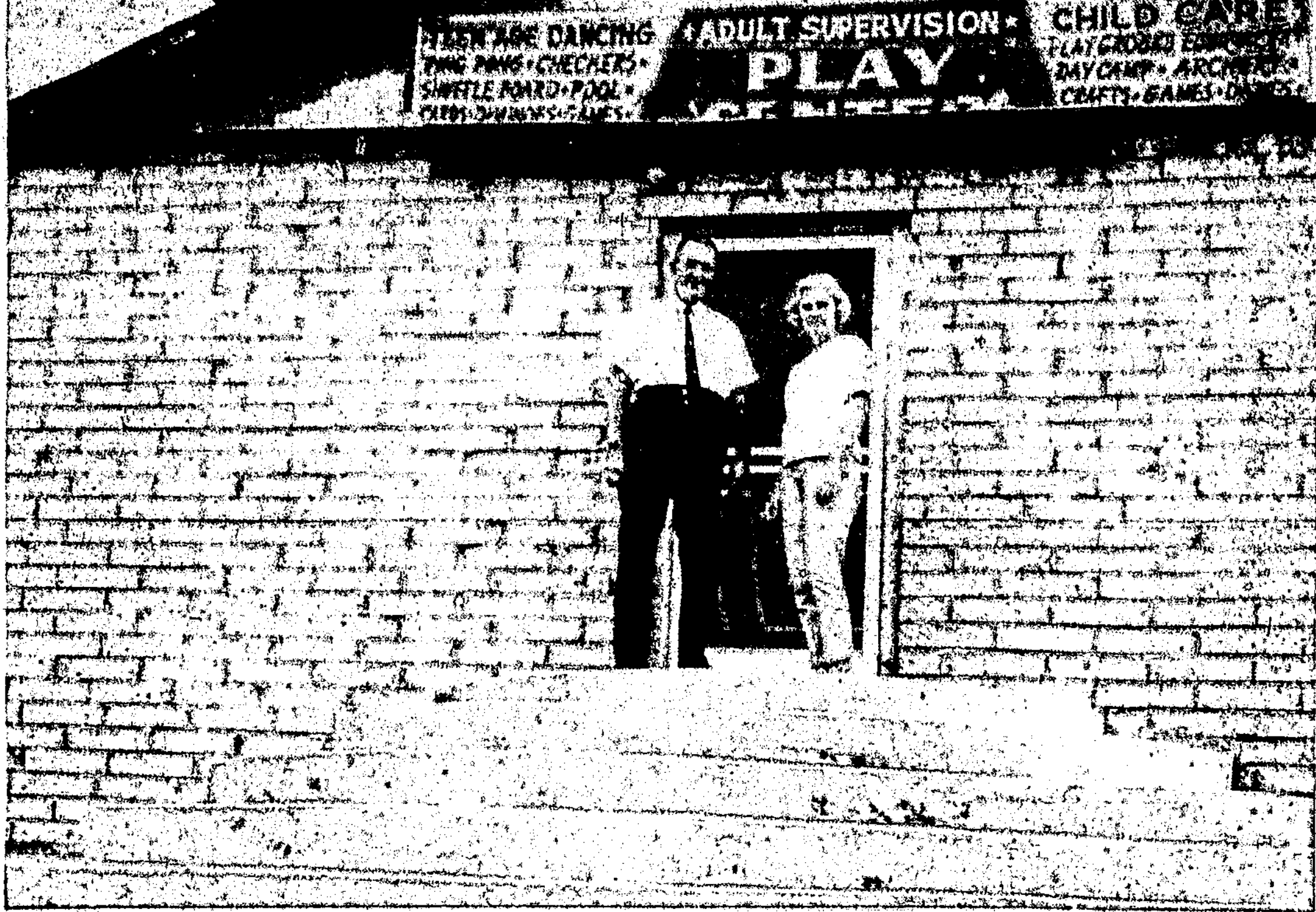
HAS NEW FRONT — Mr. and Mrs. Pete Gillespie stand on new rounded cement steps in front of their Play Center on Sudderth Drive. Brick facing was used to dress up the front.
