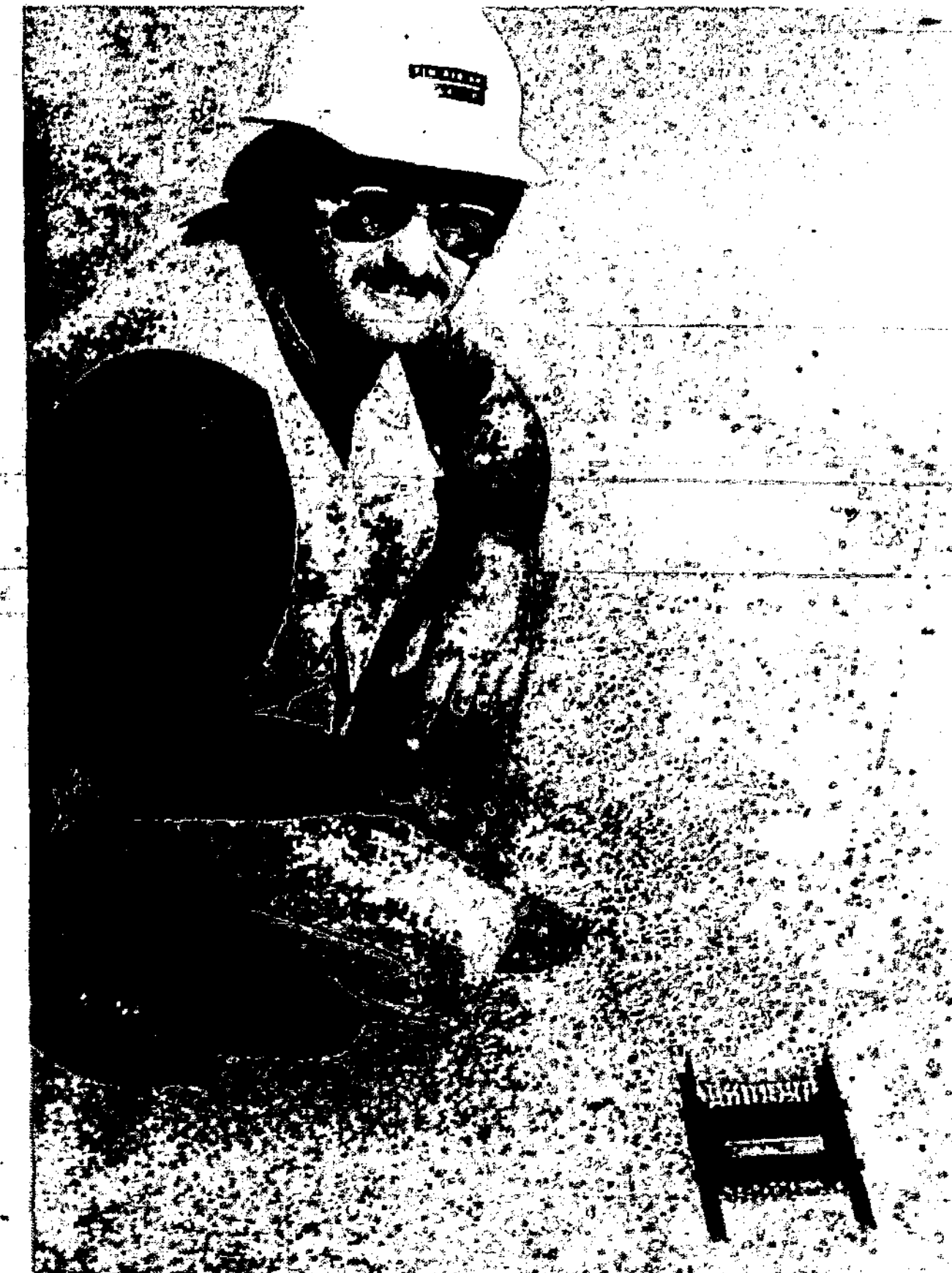
RAISED PLOWABLE MARKERS —State Highway Department Engineer Tim Basler shows an installed reflectorized marker on State Road 37. The markers are installed in three rows. An amber reflector on the markers separates opposing lanes of traffic while red and white reflectorized markers separate lanes headed in the same direction. The markers are made of cast iron with metal protectors extending above the reflectors. They are beveled on both ends to deflect snow plows. (Ruidoso News Photo)
