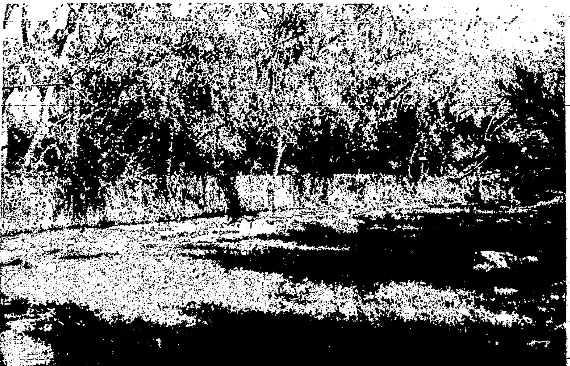
A REVETMENT of the Rio Bonito, above, has helped change the river's course through a gradual buildup of one bank. The mesh slows the velocity of the water, allowing silt to ac-
