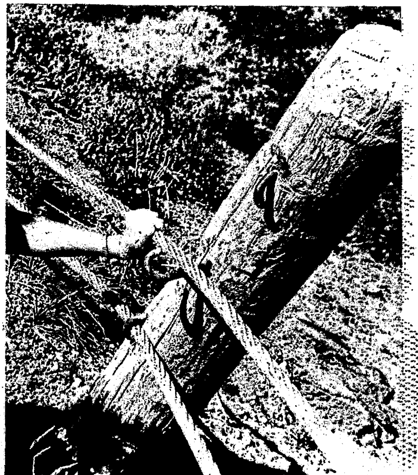
SAGGING CABLES, sometimes insecurely attached to safety posts, would seem to afford little protection to motorists traveling on State
